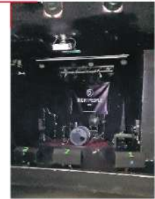
PHOTOGRAPH OF MAIN RAISED BAND AREA SHOWING RETROFIT PLASTERBOARD CEILING AND BOXING OUT OF TIMBER BEAMS. ALL PAINTED BLACK FOR NIGHTCLUB USE. FEATURE DOWNLIGHTS, ALARMS, INDICATORS AND SPRINKLERS PREDOMINANTLY SURFACE MOUNTED.
