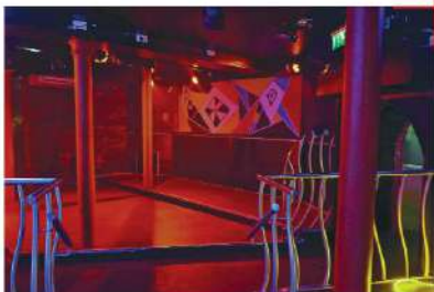
PHOTOGRAPH OF MAIN RAISED DANCEFLOOR AREA 1/021 SHOWING RETROFIT PLASTERBOARD CEILING AND BOXING OUT OF TIMBER BEAMS. ALL PAINTED BLACK FOR NIGHTCLUB USE. FEATURE DOWNLIGHTS, ALARMS, INDICATORS AND SPRINKLERS PREDOMINANTLY SURFACE MOUNTED.
