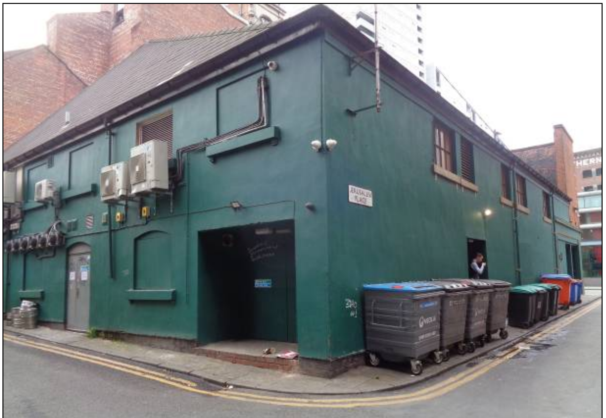
5. Side and rear elevations however retain some of the character of the original building
