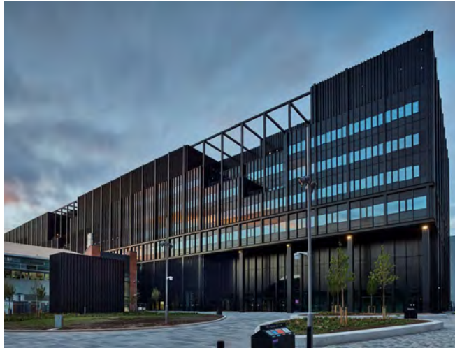
Manchester Engineering Campus Development (MECD)
