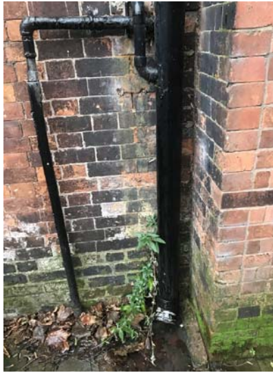
Damage to low level brick
