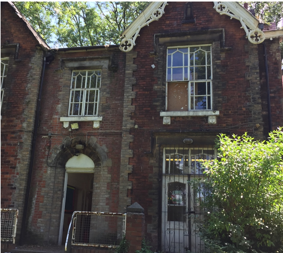
uPVC downpipes & gutters on front elevation at north-west aspect
