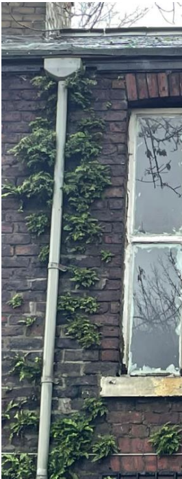
uPVC downpipe at rear elevation
