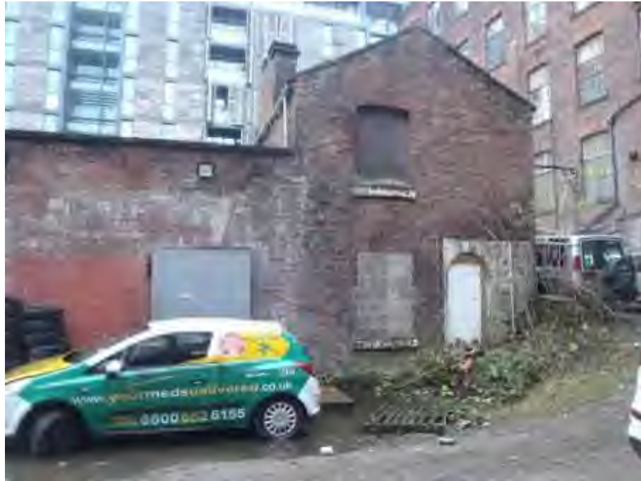
Photograph 5 – Garage and attached cottage in central courtyard, with standing water west of the garage
