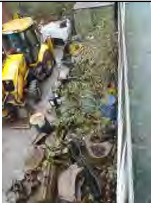
Photograph 15 – Storage yard in north-west of Site
