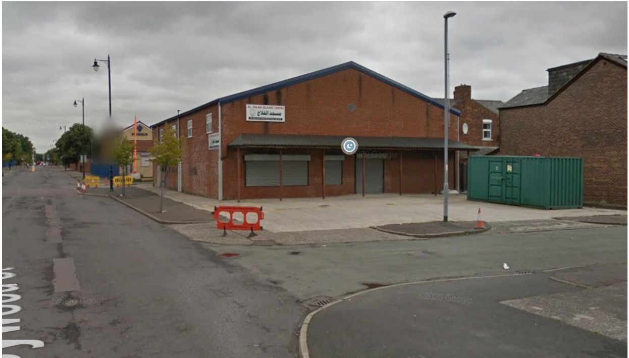
Above image shows the southern front elevation of the mosque with access and hardstanding for parking.
