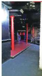
PHOTOGRAPH OF MAIN RAISED DANCEFLOOR AREA 1/021 SHOWING RETROFIT PLASTERBOARD CEILING AND BOXING OUT OF TIMBER BEAMS. ALL PAINTED BLACK FOR NIGHTCLUB USE. FEATURE DOWNLIGHTS, ALARMS, INDICATORS AND SPRINKLERS PREDOMINANTLY SURFACE MOUNTED.
