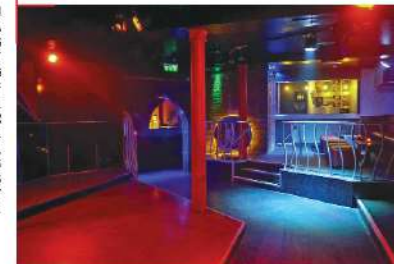
PHOTOGRAPH OF MAIN RAISED SEATING AREA AND BAR 1/022 SHOWING RETROFIT PLASTERBOARD CEILING AND BOXING OUT OF TIMBER BEAMS. ALL PAINTED BLACK FOR NIGHTCLUB USE. FEATURE DOWNLIGHTS, ALARMS, INDICATORS AND SPRINKLERS PREDOMINANTLY SURFACE MOUNTED.
