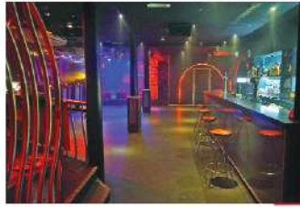
PHOTOGRAPH OF MAIN BAR AREA 1/005 SHOWING RETROFIT PLASTERBOARD CEILING AND BOXING OUT OF TIMBER BEAMS. ALL PAINTED BLACK FOR NIGHTCLUB USE. FEATURE DOWNLIGHTS, ALARMS, INDICATORS AND SPRINKLERS PREDOMINANTLY SURFACE MOUNTED.
