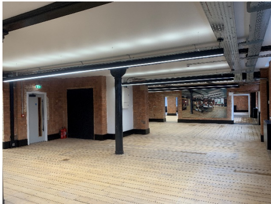
Figure 5: Looking south from Unit 01 into Unit 02 showing the location of the proposed stud partition to divide the two units.
