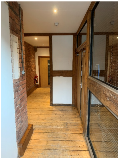
Figure 22: The lobby as seen from the recently completed link bridge, showing the modern, faux-timber framing forming a partitioned corridor.
