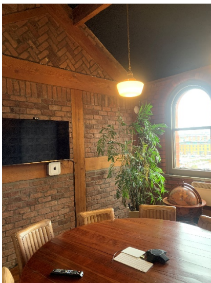
Figure 18: An example of a meeting room to the centre of the unit, showing the modern faux-timber-framing and brickwork beneath the original exposed roof structure.
