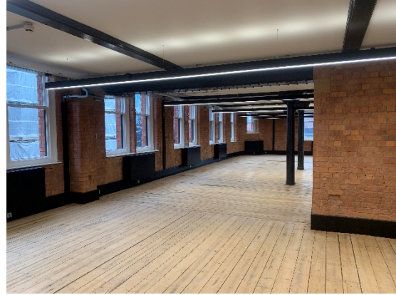
Figure 4: Looking north from Unit 02 into Unit 01, showing the location of the proposed stud partition within to divide the two units.
