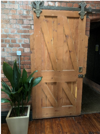
Figure 16: An example of one of two original surviving pitch pine roller fire doors to the top of the former landing.
