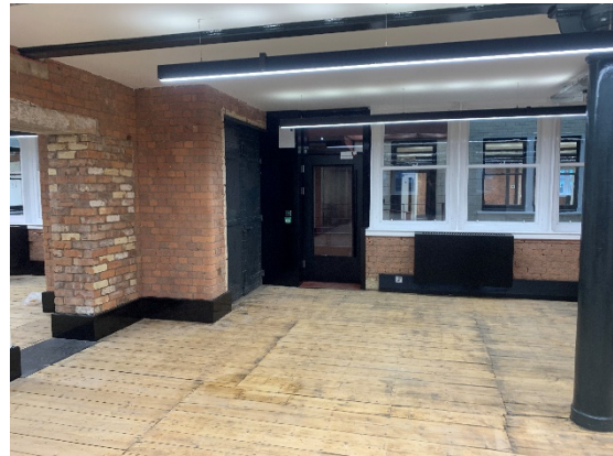
Figure 6: One of the new entrances into Unit 01 from the central lightwell.
