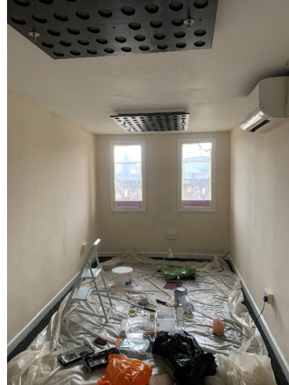
Figure 13: Looking into one of the two former sound-insulated studios, showing the independent internal lining of the studio and the two modern openings looking into the original windows behind.
