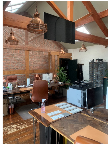
Figure 21: An example of the original exposed roof structure and modern brick and timber-framing insertion beneath.
