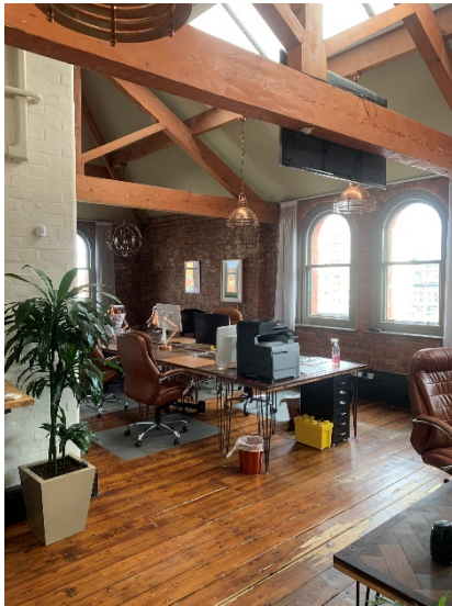
Figure 20: The northern half of the unit, showing the exposed original floorboards and roof structure.
