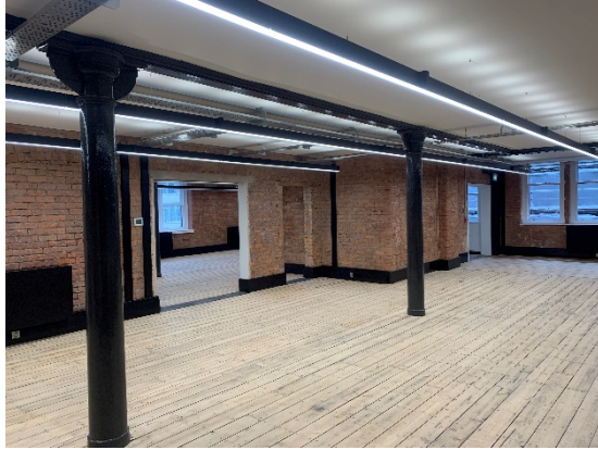
Figure 3: Looking west across Unit 02.
