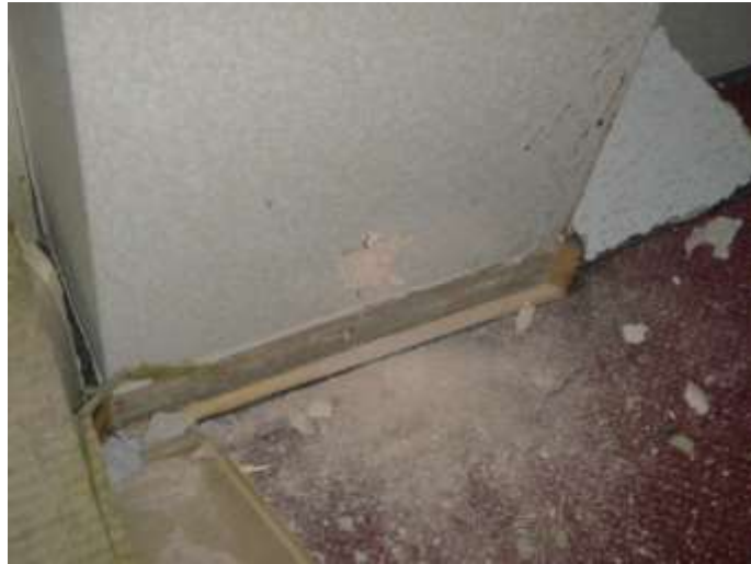
Concrete and Plaster with Timber Skirting to Base of Column C3
