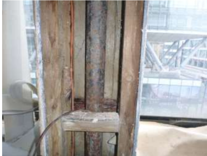
Timber and Plaster Boxing to Column C6
