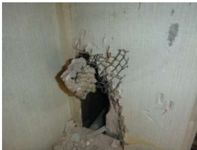
Mesh and Plaster to Base of Column C4
