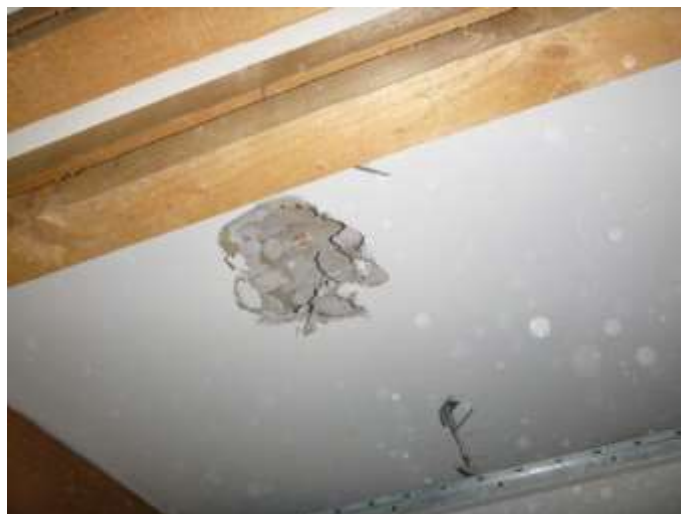
Plasterboard to Ceilings below L02 Slab
