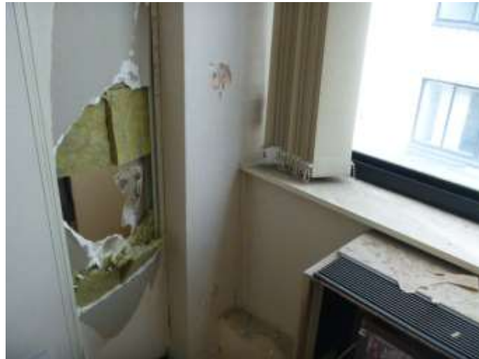
Concrete and Plaster to Column C7 (Plasterboard and Rockwool to Partition)
