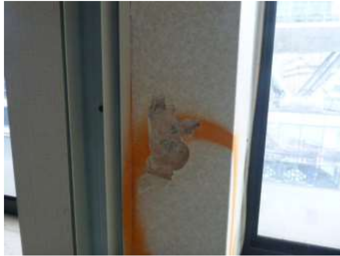
Plaster to Column C1
