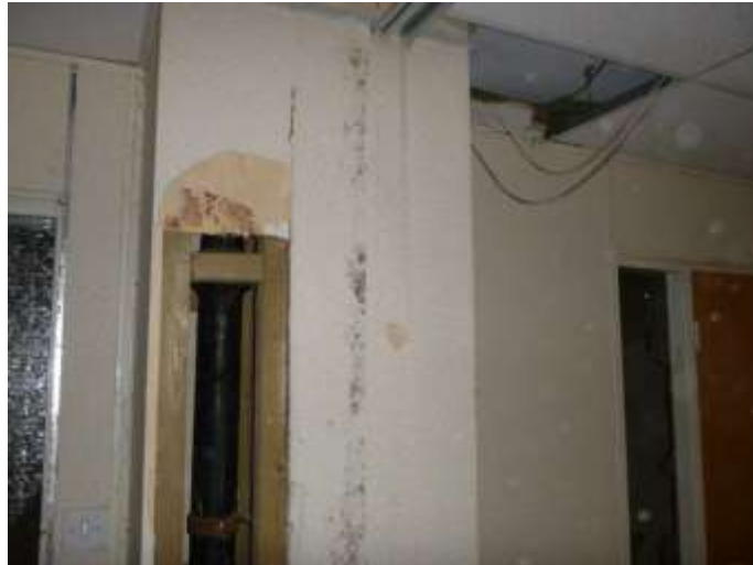
Timber Boxing to side of Column C8
