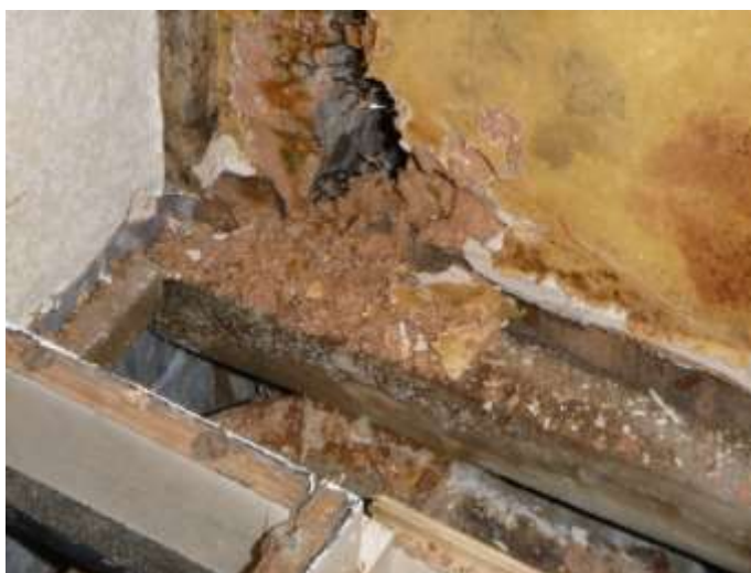
Mesh and Plaster with Timber Boxing to Base of Column C6
