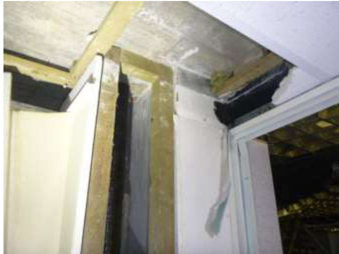
Timber Boxing to Column C5
