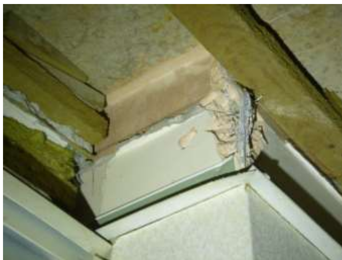
Rockwool and Timber to Top of Column C3
