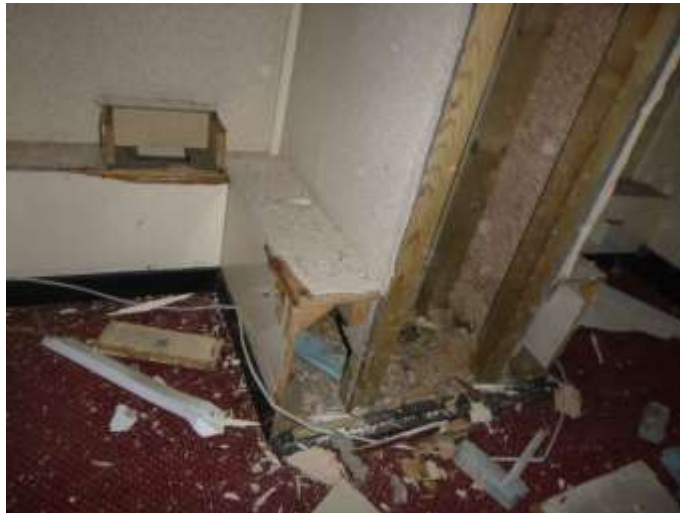
Timber Boxing to Base of Column C2
