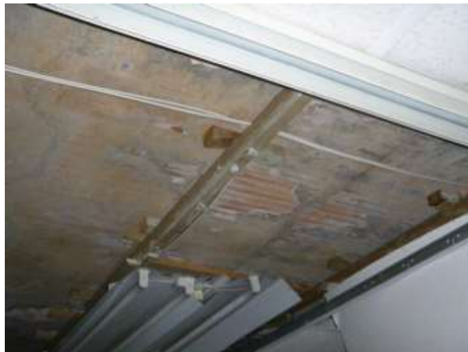
Pot and Beam to L03 Slab
