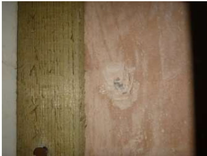
Plaster over Concrete to Column C3
