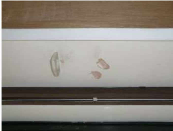
Plaster to Beams above Windows
