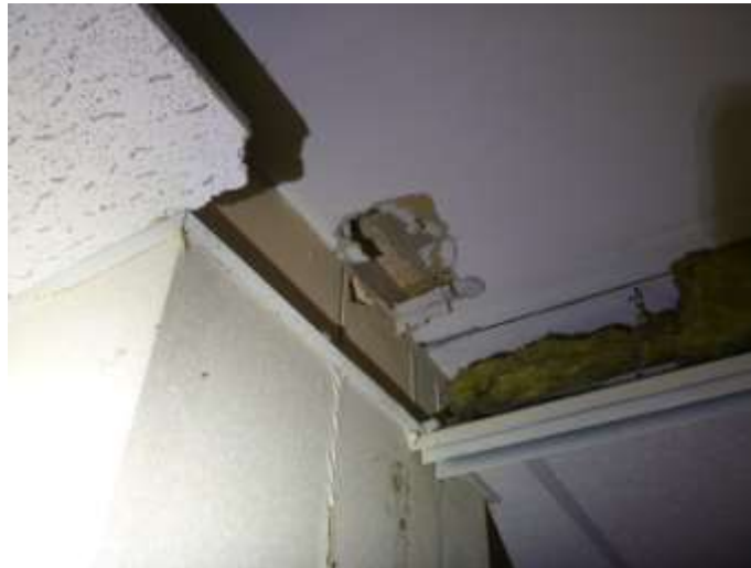
Plasterboard to Ceiling at Top of Column C7
