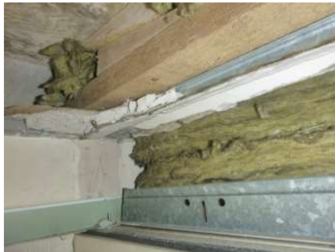
Plasterboard and Rockwool adjacent to the Top of Column C1
