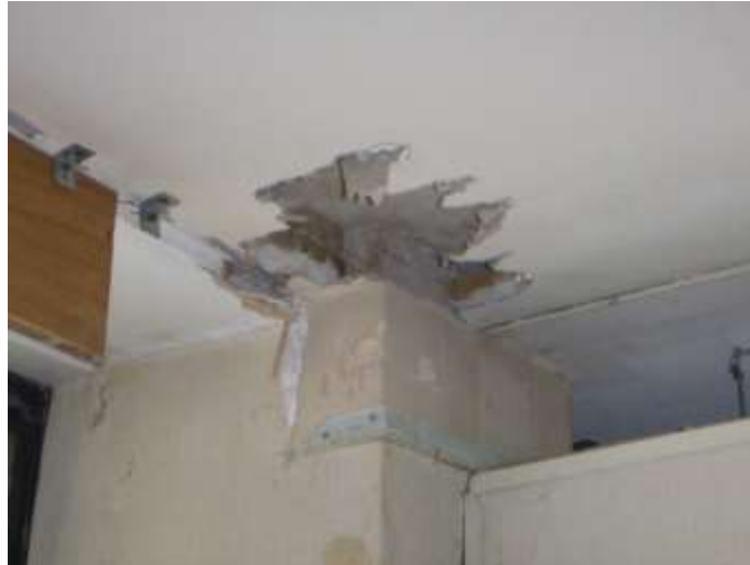
Concrete and Plaster to Top of Column C6
