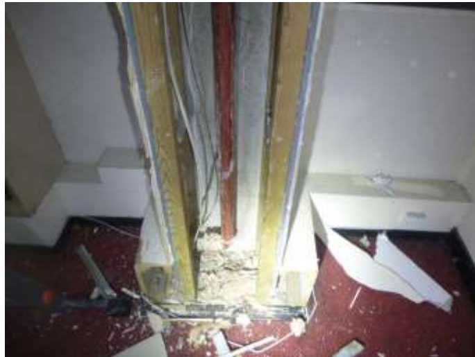
Timber with Mesh and Plaster to Front of Column C2
