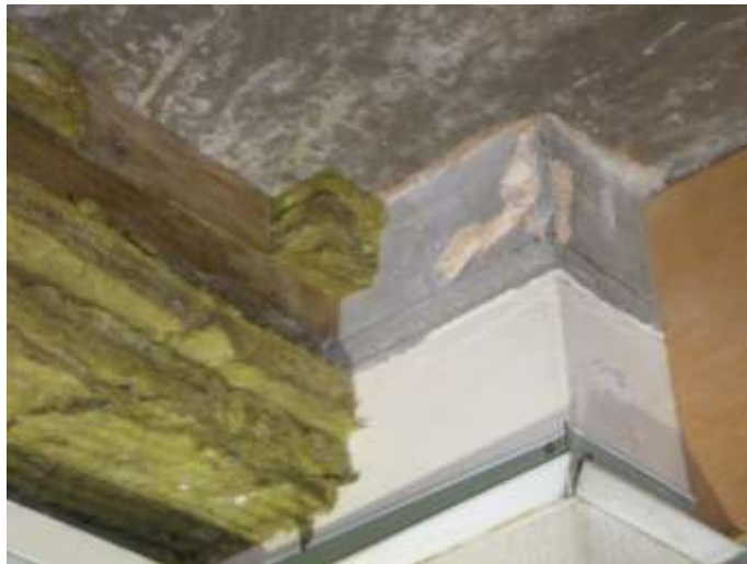
Concrete and Plaster to Top of Column C4
