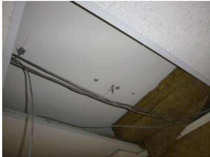
Plasterboard to Ceilings below L02 Slab
