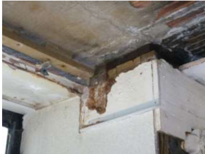
Plaster to Beam and Timber Boxing to Top of Column C6
