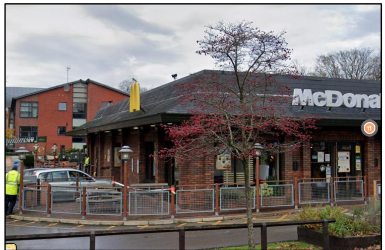
Figure 16: Outdoor eating/drinking area to Mc Donalds at 336 Wilmslow Road.
