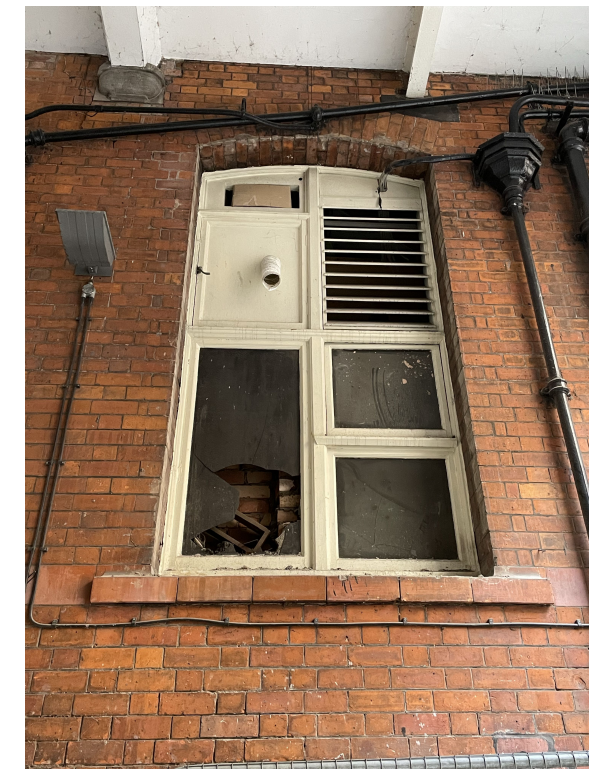
Photograph of existing window 31/03/22
