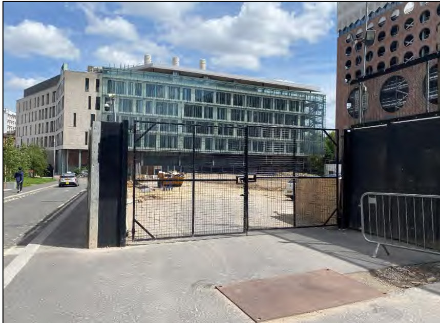
Figure 3.2 – Existing Site Frontage, Viewed from Newman Street Eastbound
