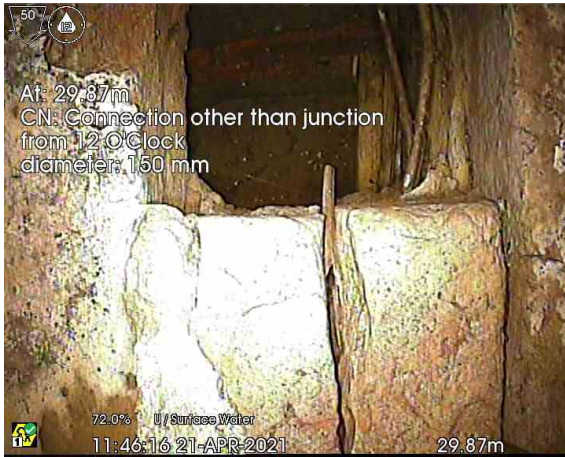
2_29-87m_114616.jpg, 00:07:01, 29.87 m Connection other than junction at 12 o'clock, diameter: 150mm
