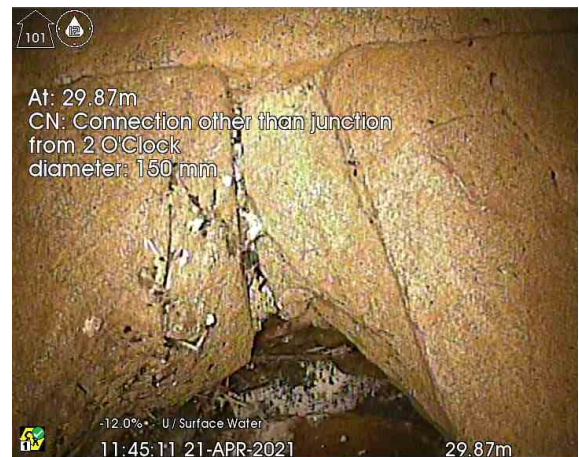
2_29-87m_114511.jpg, 00:06:07, 29.87 m Connection other than junction at 2 o'clock, diameter: 150mm
