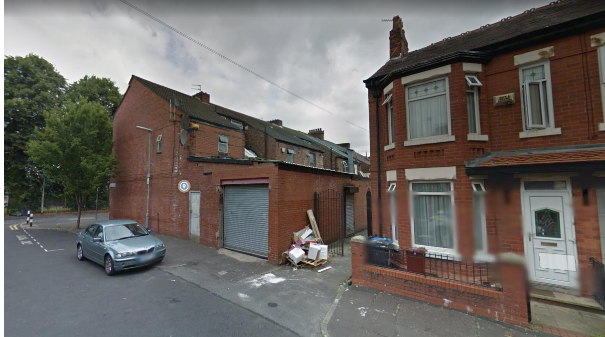
The above image shows the context of the site when viewed to the North on Spencer Avenue
