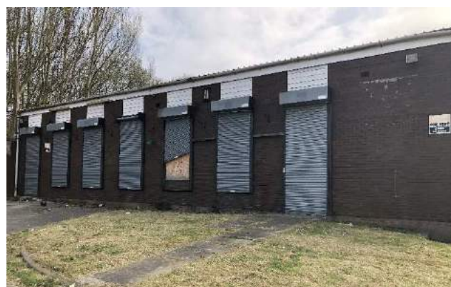
Photo 6: Building- western side.
