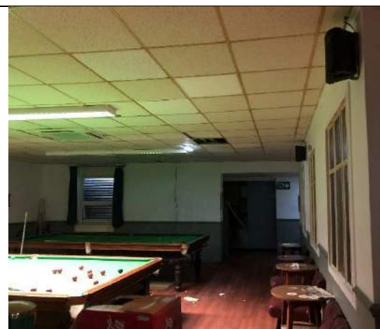
Photo 16: Bar and pool area east side of building. Holes in roof, inspected and noted unsuitable for bats.
