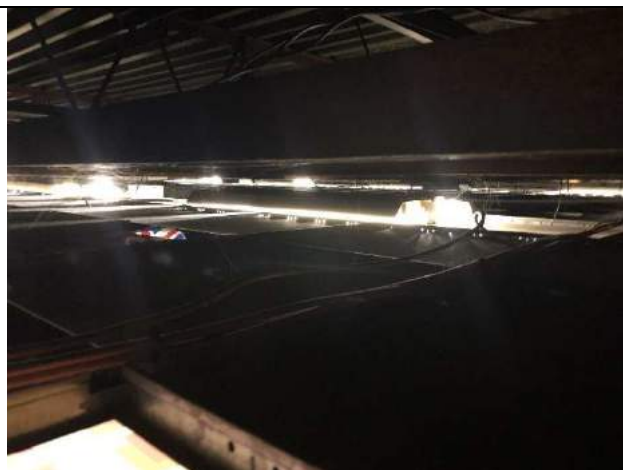
Photo 14: Suspended ceiling above large dance hall, west side of building.
