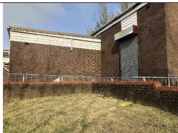
Photo 8: Building - east side
