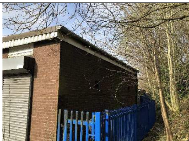
Photo 9: Building – north side. Unable to be surveyed due to fence and dense scrub.
