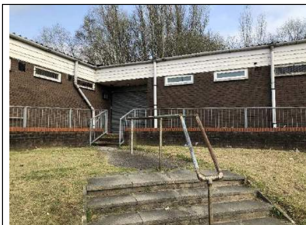
Photo 7: Entrance to building - south east side
