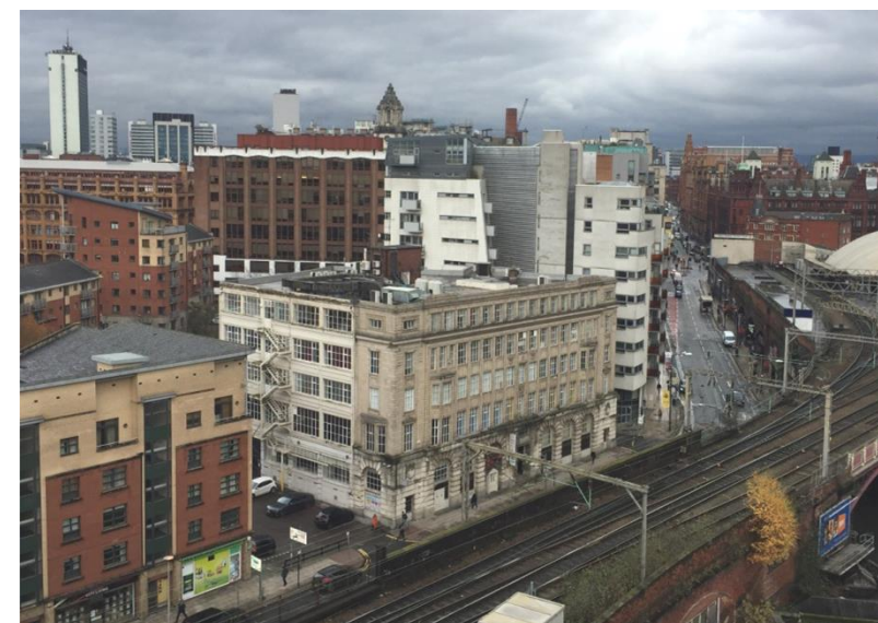
General view of Barclay House
