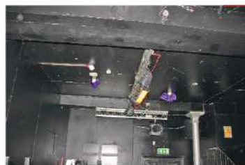
PHOTOGRAPH OF SEATING AREA 0/010 SHOWING RETROFIT PLASTERBOARD CEILING AND BOXING OUT OF TIMBER BEAMS. ALL PAINTED BLACK FOR NIGHTCLUB USE. LIGHTS, ALARMS, INDICATORS AND SPRINKLERS PREDOMINANTLY SURFACE MOUNTED.
