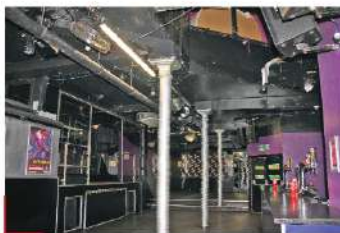
PHOTOGRAPH OF SEATING AREA 0/003 SHOWING RETROFIT PLASTERBOARD CEILING AND BOXING OUT OF TIMBER BEAMS. ALL PAINTED BLACK FOR NIGHTCLUB USE. LIGHTS, ALARMS, INDICATORS AND SPRINKLERS PREDOMINANTLY SURFACE MOUNTED.
