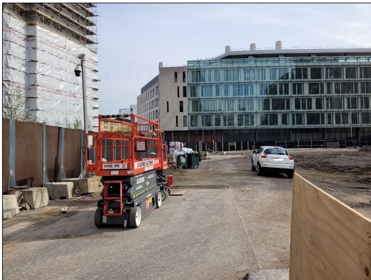
Photograph 1 Recently cleared area of the site
