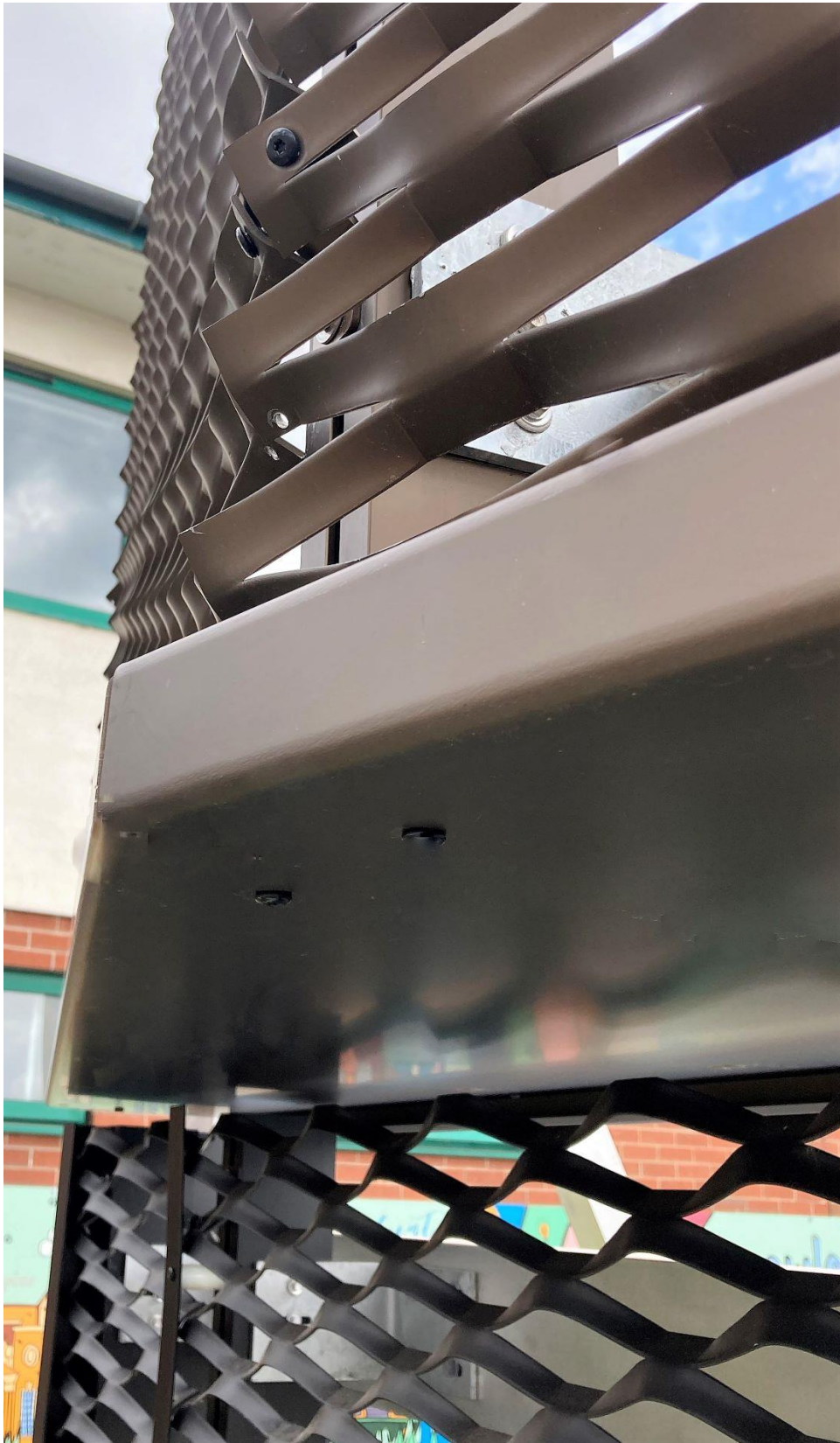
Level 01 Flashing Detail
