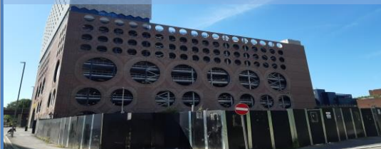
The site, partly enclosed with tall hoardings, and the Premier Inn and MSCP behind
