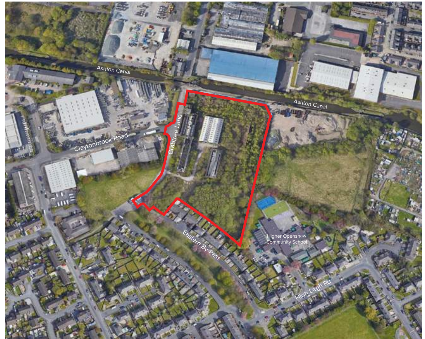
Aerial view of the site, with application site boundary edged in red.
