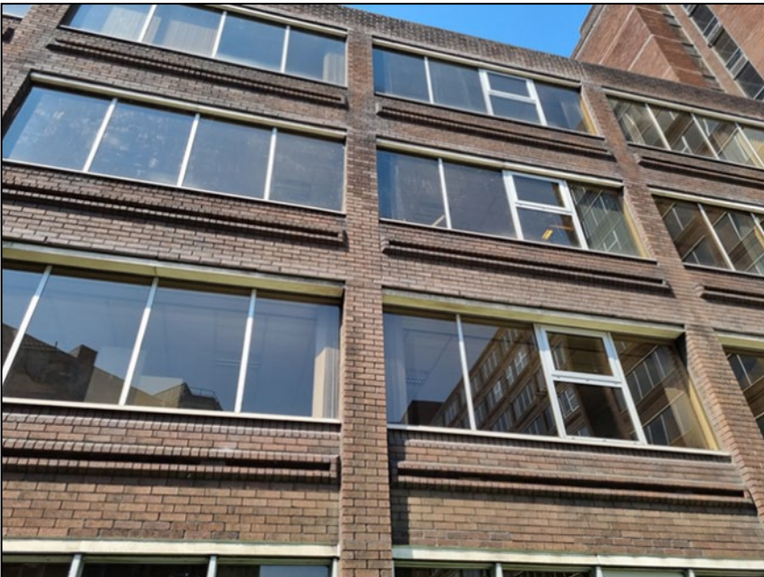
Photo 7 Masonry in good condition and no gaps around window frames
