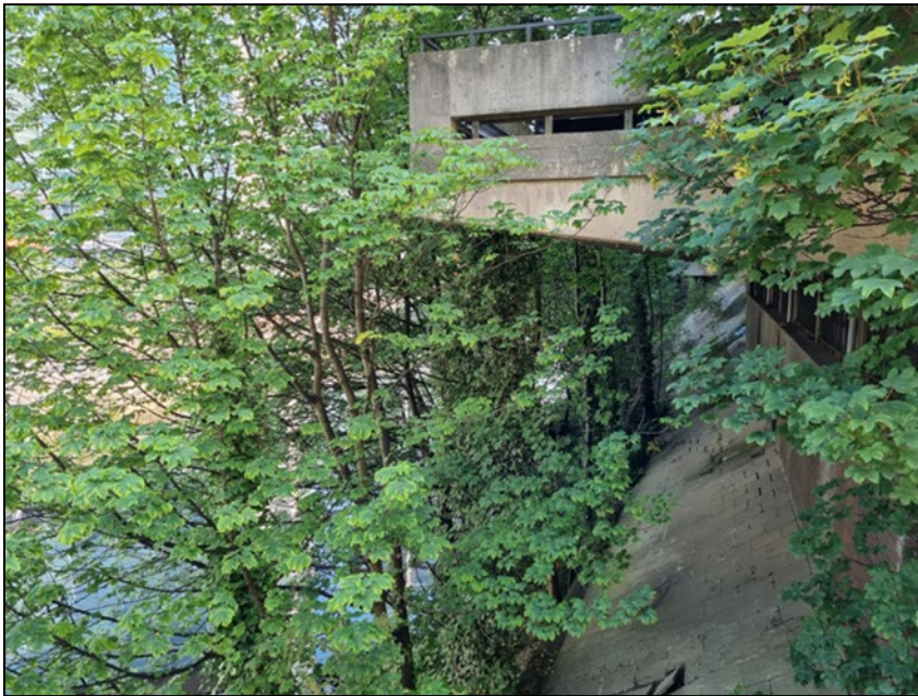
Photo 4 Balcony at rear of building
