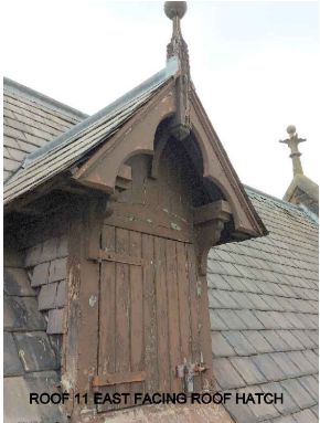
1 Photo of East facing roof hatch NTS
