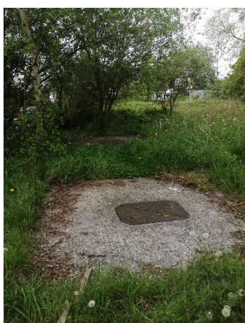
Photo 11: Hard standing with manhole covers present on site.
