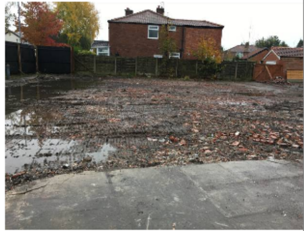
Photo 2: View of site post demolition looking southeast.
