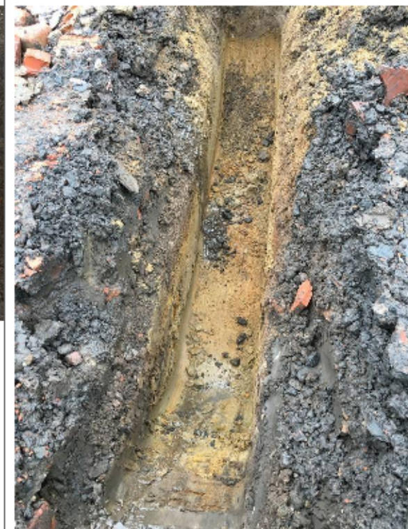
Photo 7: Trial Pit 3. Some perched water in Made Ground flowing into pit to left of photo. Made Ground over Glaciofluvial sand.
