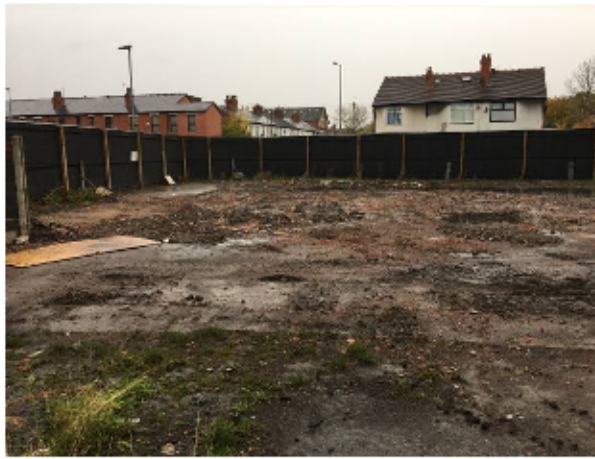
Photo 1: View of site post demolition looking northwards, towards School Lane.
