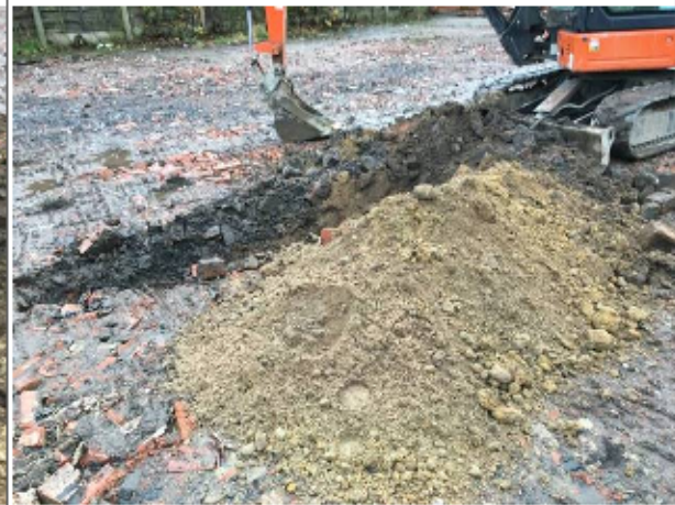
Photo 5: Trial Pit 2. Close up of excavated natural Glaciofluvial sand.
