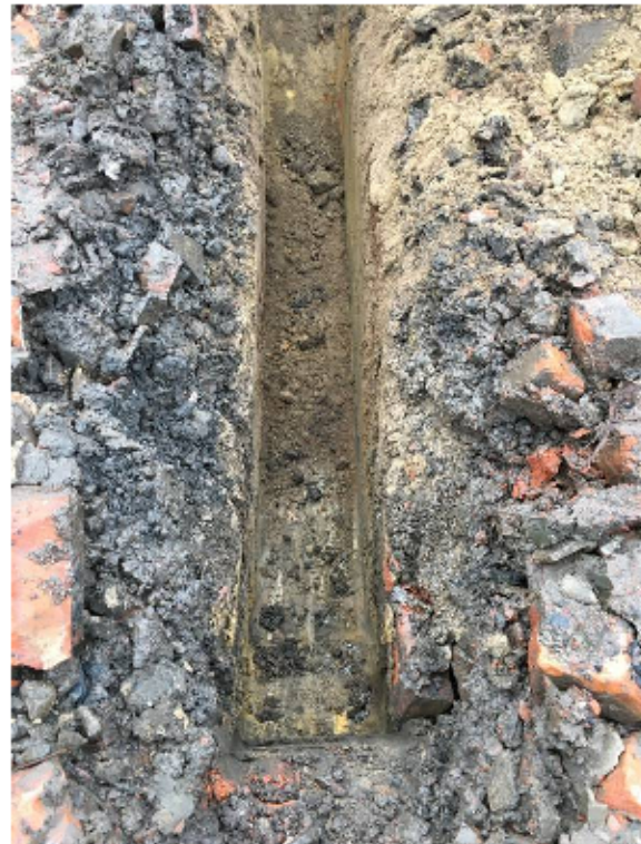
Photo 3: Trial Pit 2. Showing Made Ground over natural Glaciofluvial sand.
