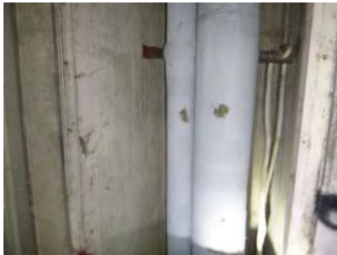
Rockwool Pipe Insulation to Stairs Risers
