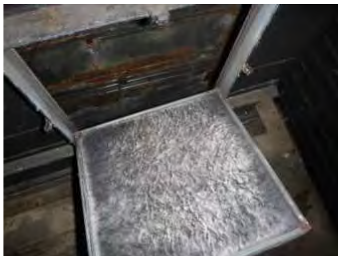
Modern Insulation to Metal Vents
