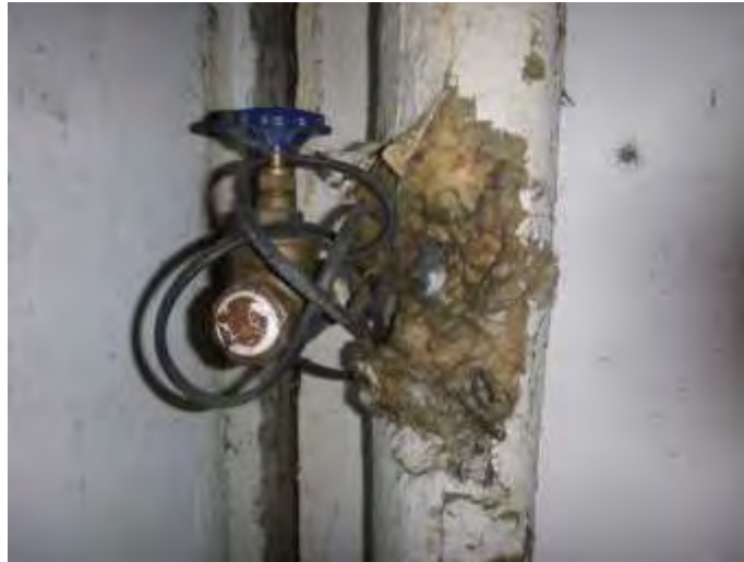
Rockwool Pipe Insulation to Pipe on Mid-Level
