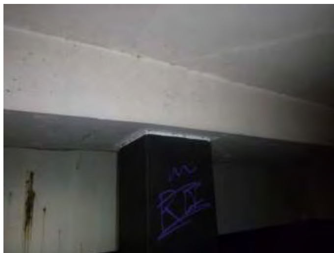
Concrete Columns and Beams
