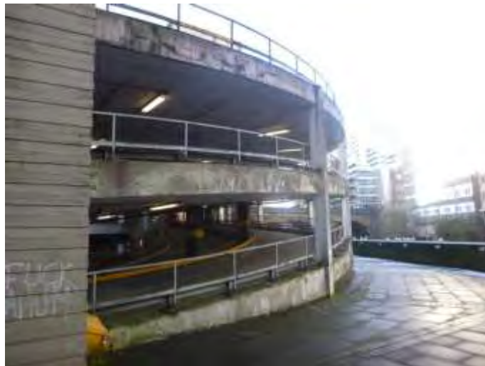
Concrete Vehicle Ramp
