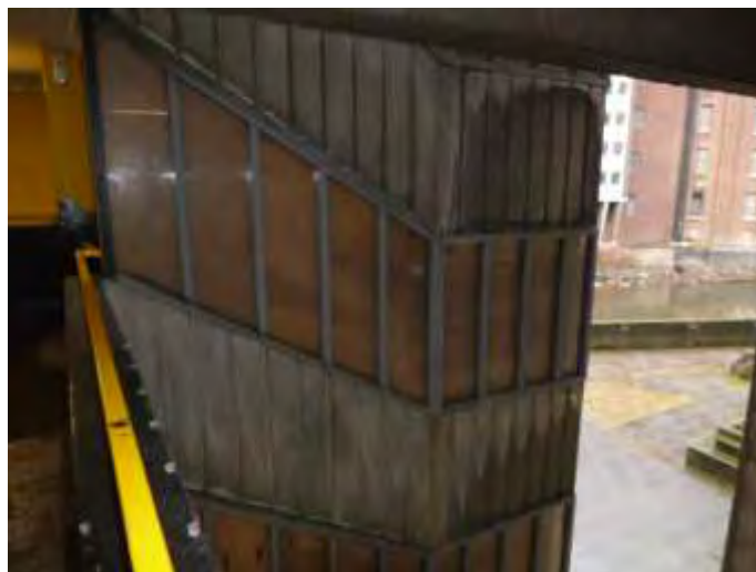
Timber behind Glazed Panels to Stairwell
