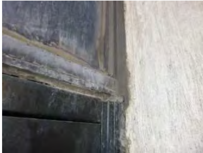
Modern Sealant to Door Panel on Exterior Lower Wall
