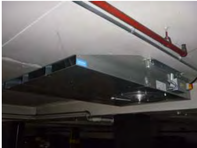
New Vent Installation
