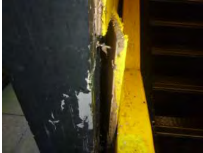
Timber Lining to Stairs Wall Panels (front stairwell)
