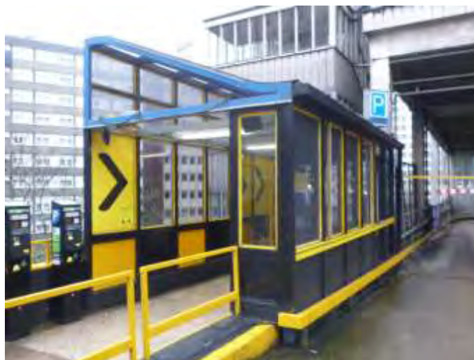
Steel / Glazed Entrance Walkway
