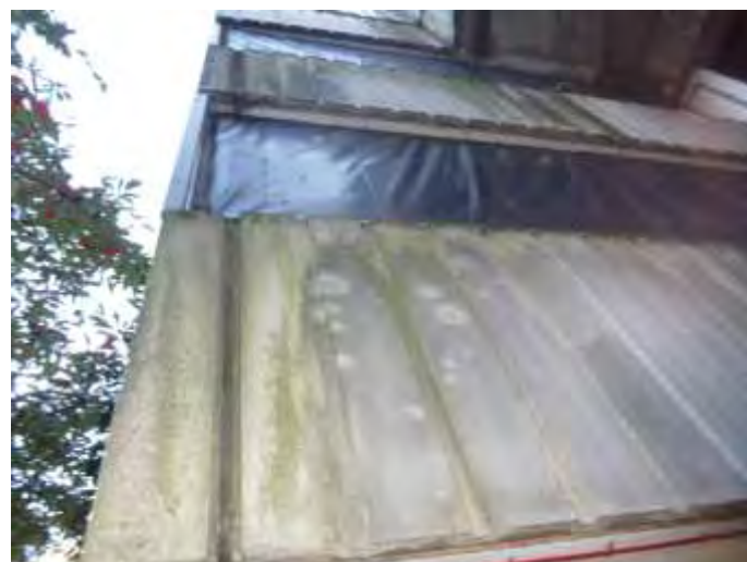
Concrete Walls and Plastic to Stairwells
