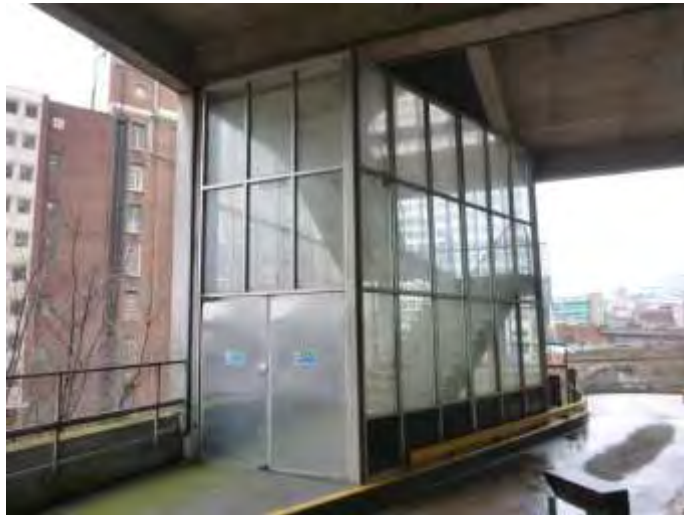
Steel Glazed Panels to Concrete Stairs near Vehicle Entrance
