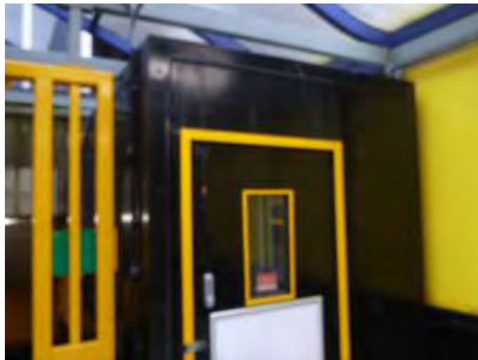
Steel and Timber Cabin adjacent to Main Entrance
