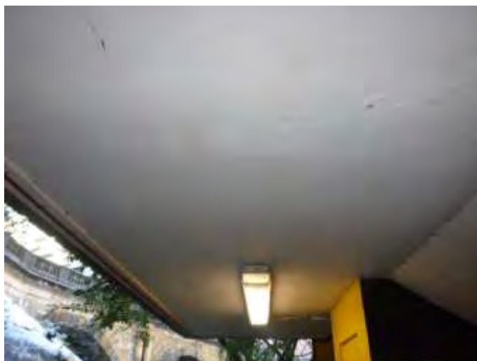
Concrete Ceilings to Stairwells
