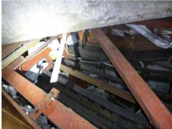
Steel Disused Escalator (only underneath accessible)
