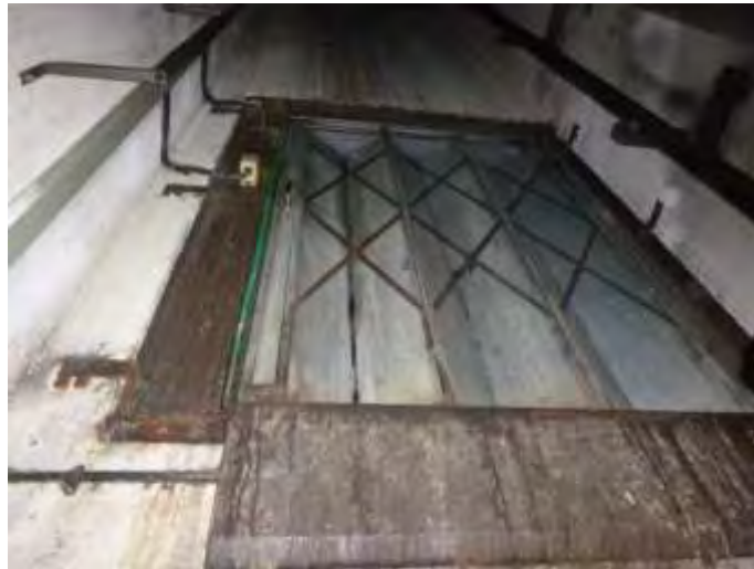
Concrete Lift Shaft and Steel Doors to Hotel Laundry Lift
