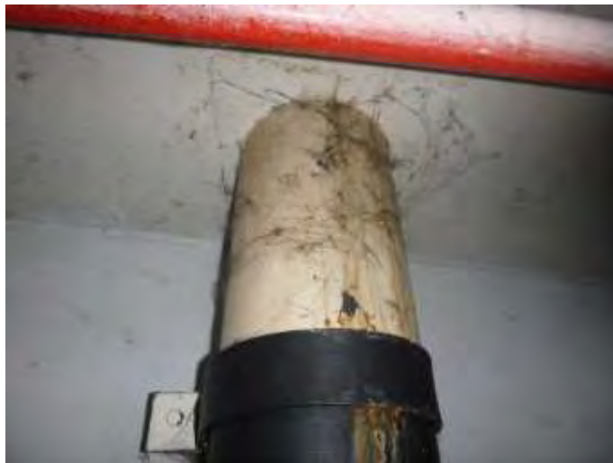
Cast Pipes from Upper Levels
