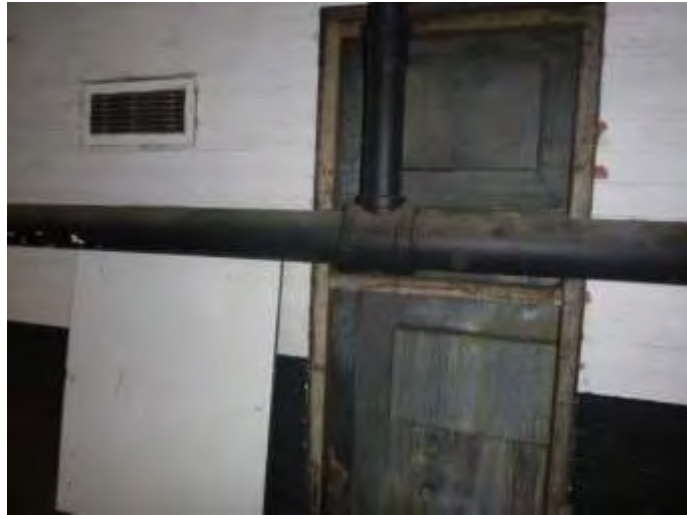
Steel Vent / Ducts behind Timber Panels to Rear Wall (Lower Level)
