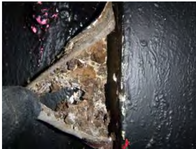
Cork behind Modern Sealant to Concrete Joints
