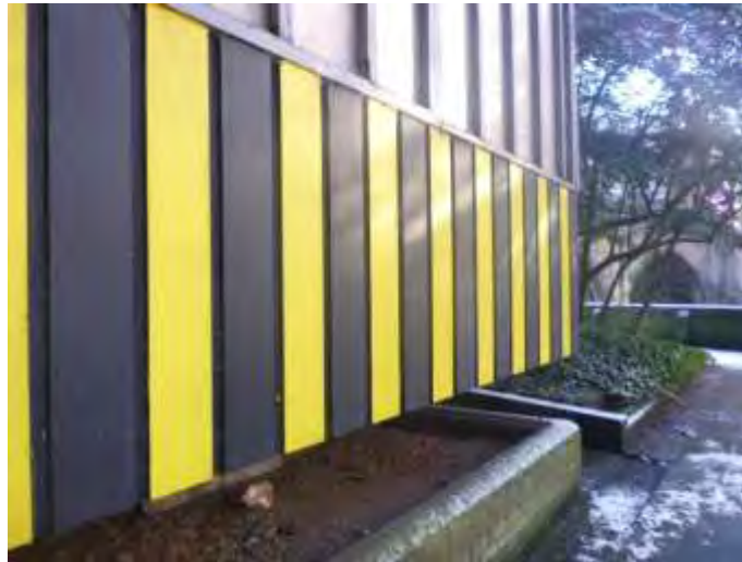
Concrete Exterior Wall to Lower Level
