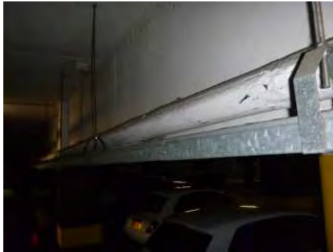
Rockwool Insulation to Pipe along Beam on Upper Level
