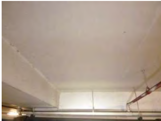
Concrete Decks to Upper Levels
