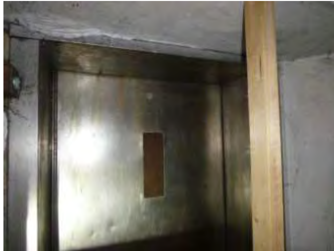
Steel Doors and Surrounds to Disused Pedestrian Lift
