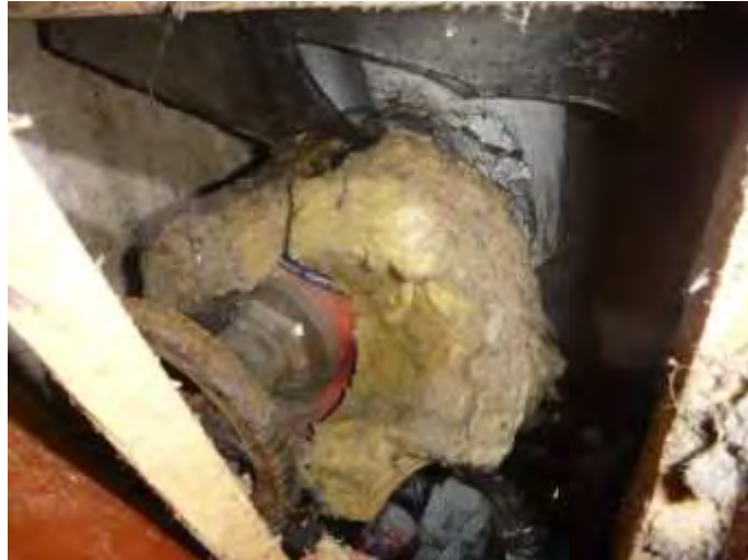
Rockwool Insulation to Risers in Stairwells
