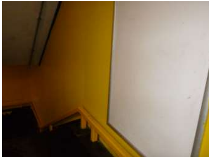
Timber Lining to Stairs near Main Entrance
