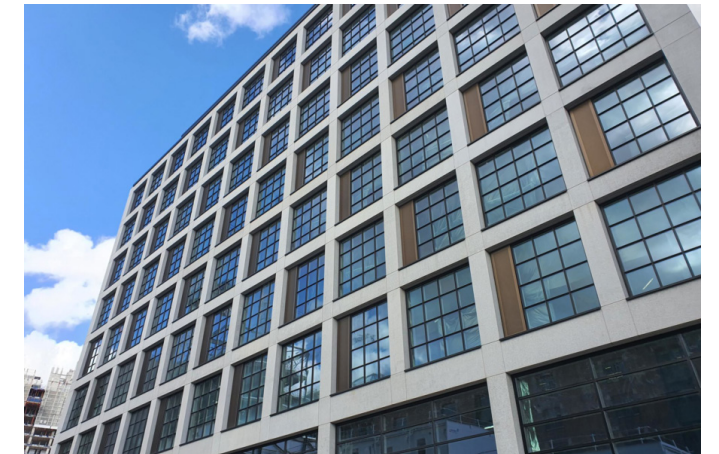
MANCHESTER GOODS YARD
