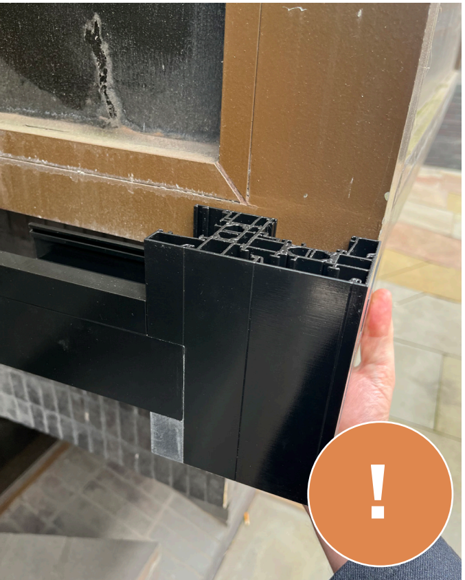
Return vertical has a design tolerance to accommodate a new fully insulated system c.7mm
