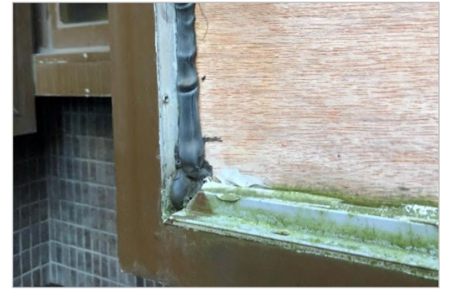
Photograph No. 27 – Timber panel installed, and silicone sealed around the jamb edges (Level 1 – North elevation – King Street Block)
