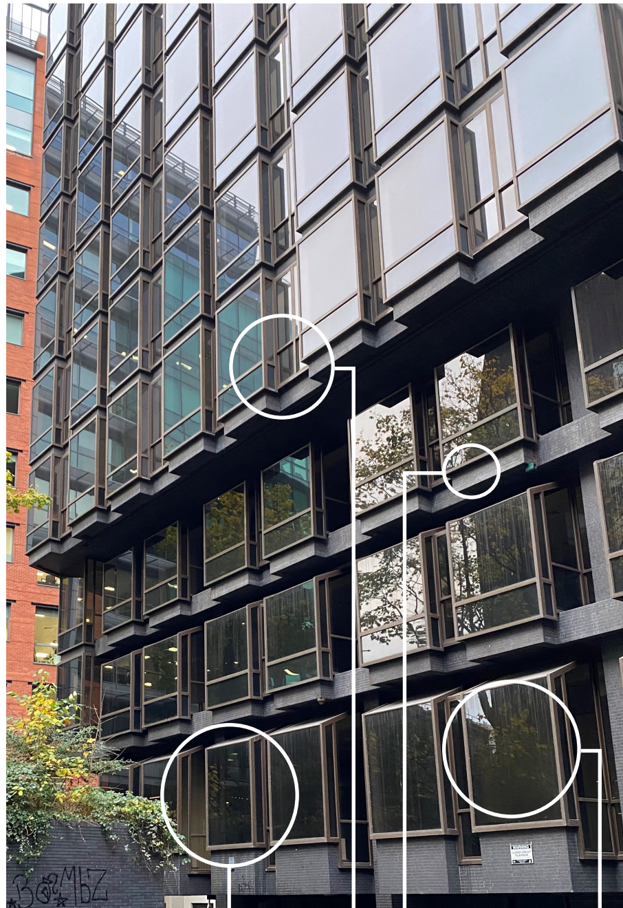
Photograph No. 15 – Paintwork deteriorated on top of framework (Level 6 – West elevation – Pall Mall Court)
