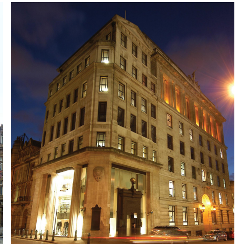
03 - SHIP CANAL HOUSE
