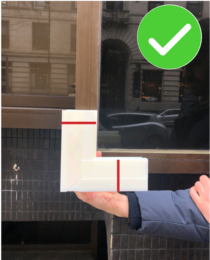
Dimensional consistency of overall build up
