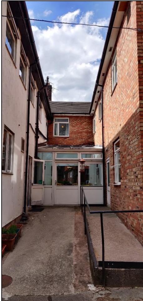
Photograph 11 showing part of the roof of the building
