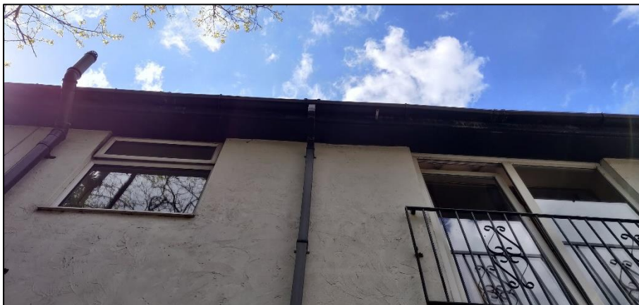
Photograph 10 showing the soffits
