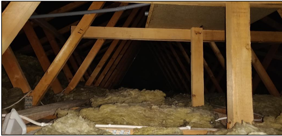
Photograph 15 showing one of the newer loft voids and timbers
