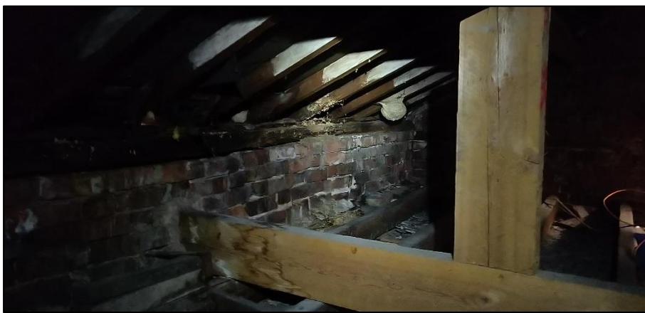
Photograph 13 showing the timbers within one of the voids
