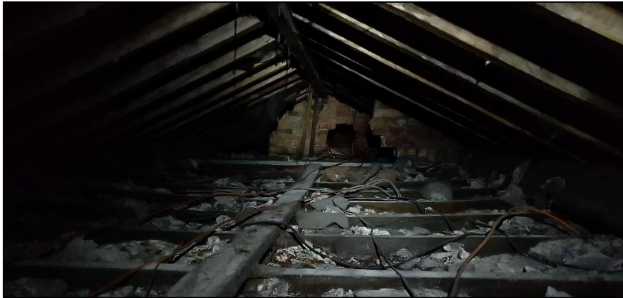
Photograph 12 showing one of the loft voids
