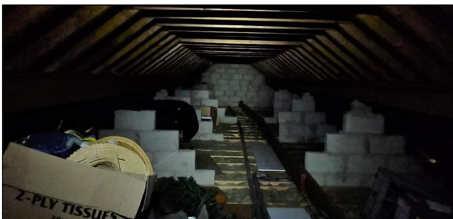
Photograph 14 showing one of the loft voids within the extensions
