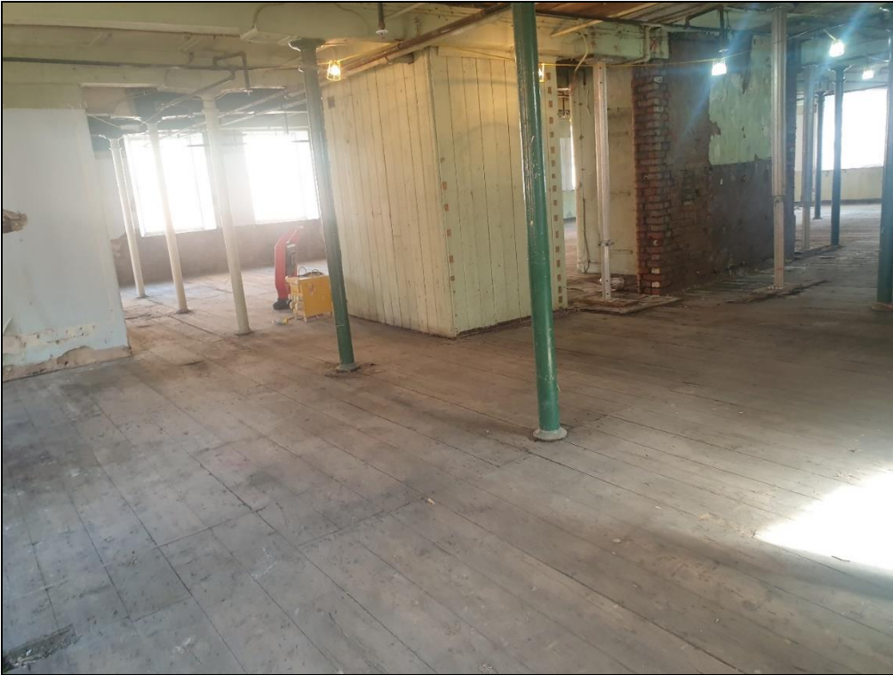
Example of timber panelling found around lift on third floor
