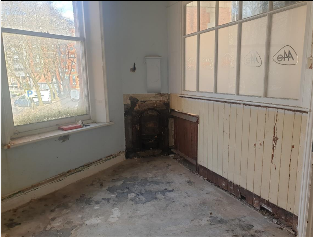
Timber panelling up to revealed fireplace floor
