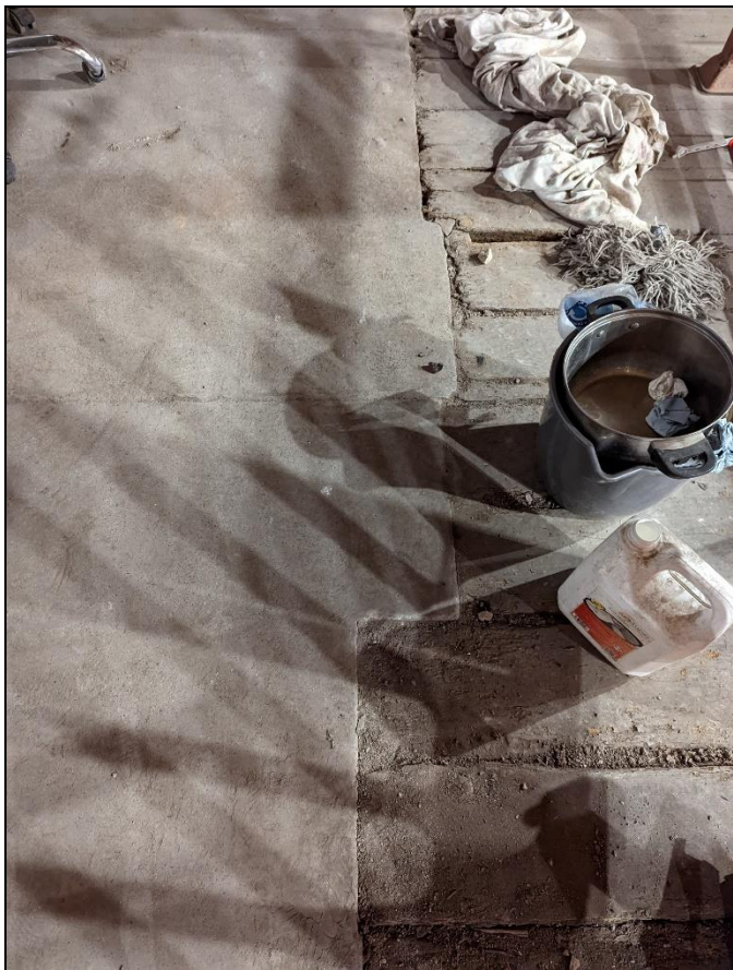
Line of concrete butting against timber boards evocative of flag stones
