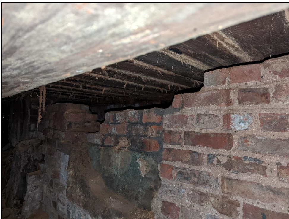
Brick wall supporting boards at junction with concrete, showing a pink lime mortar suggestive of 19 th century construction
