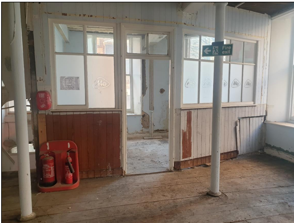
Timber panelling forming office of first floor
