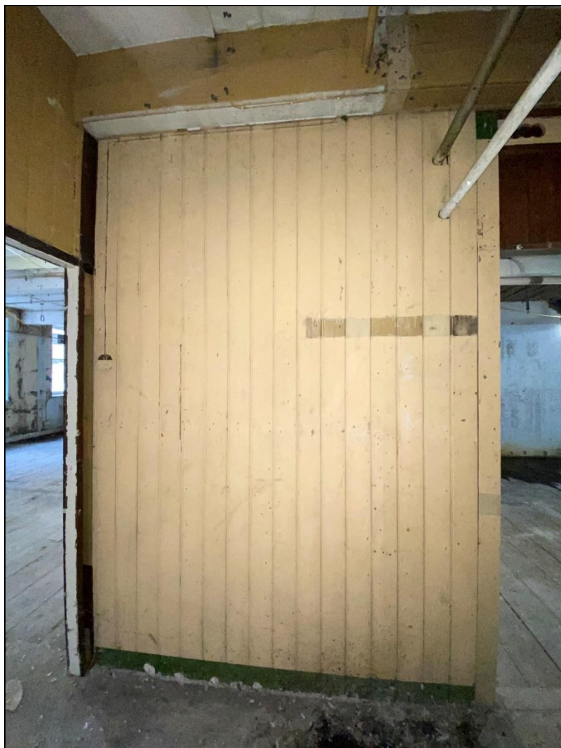
Example of timber panelling found on third floor
