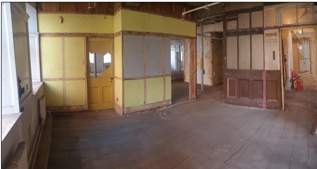
Panelling / partitions on second floor
