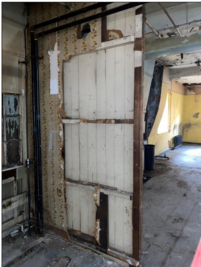
Timber partition / panelling at fourth floor.
