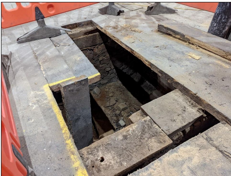
Boards supported on stone walls
