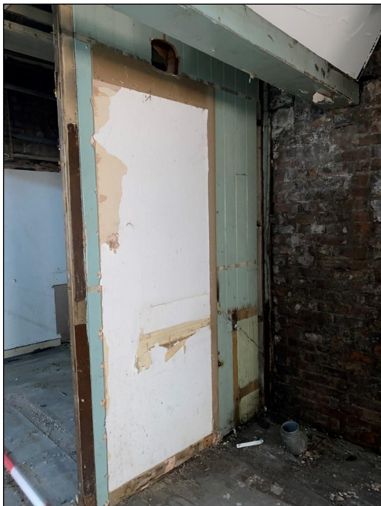
Timber partition / panelling at fourth floor.
