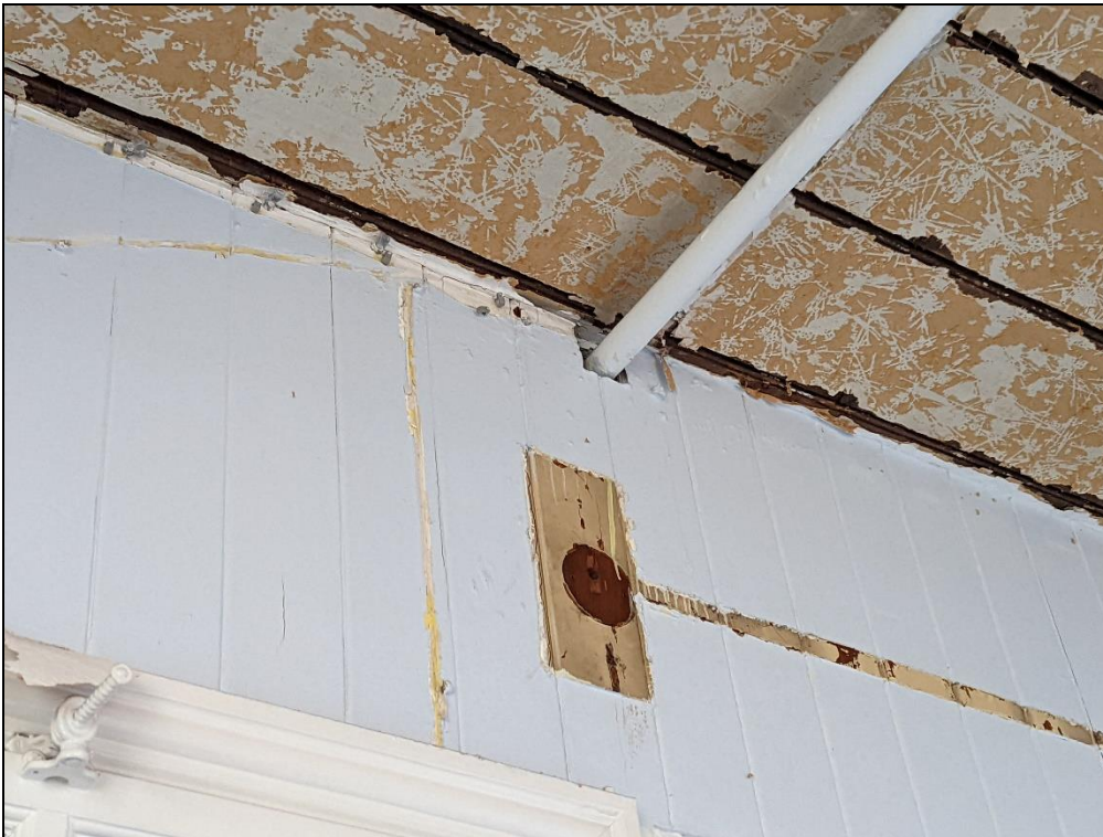
Timber panelling cut around sprinkler system
