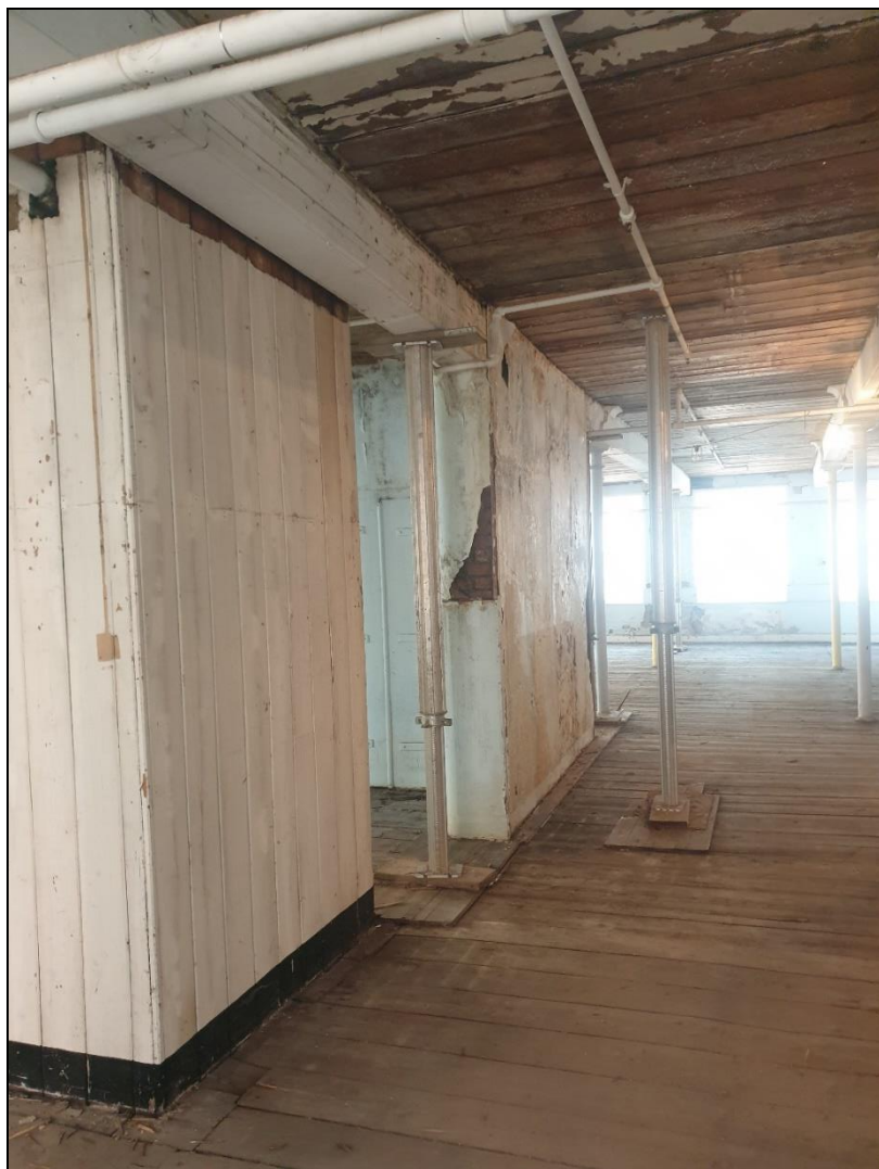
Example of timber panelling found on first floor
