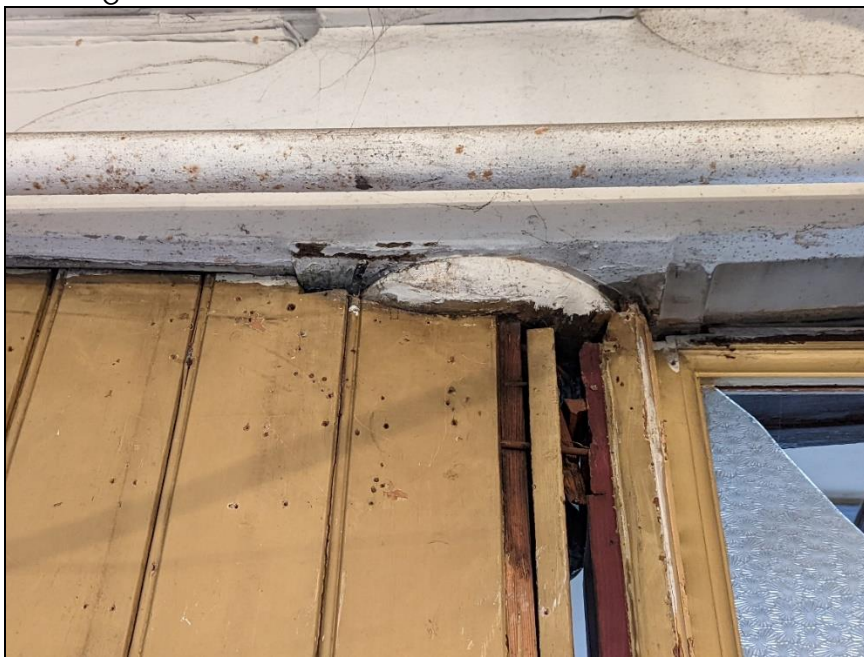
Crude panelling installation detail around stanchion
