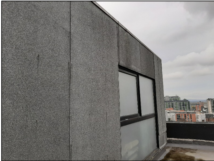
Photograph 3 – structure to be demolished
