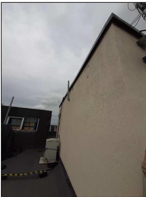
Photograph 7 – service lift building that may be disturbed
