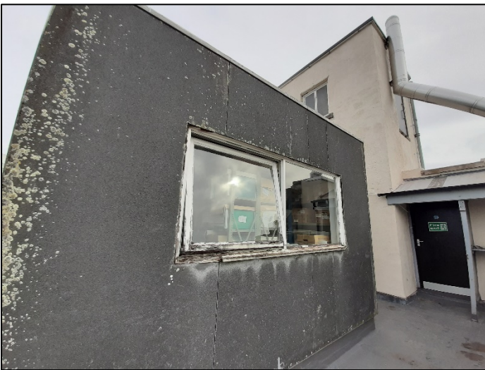
Photograph 2 – structure to be demolished
