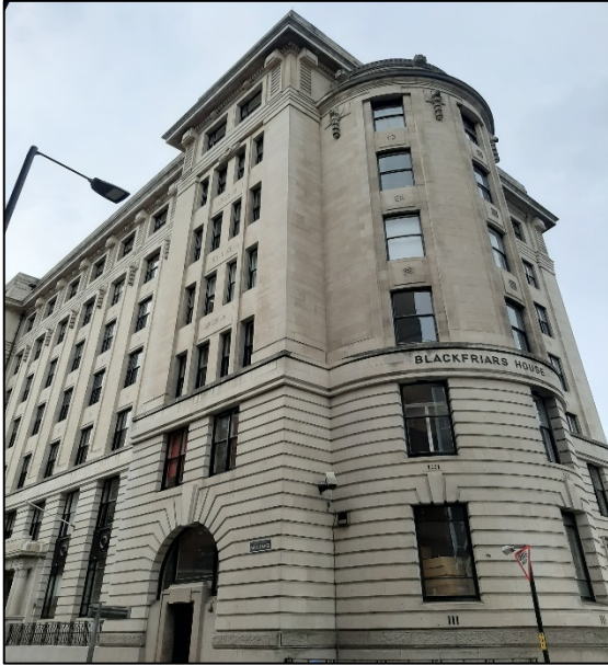
Photograph 1 – exterior of Blackfriars House
