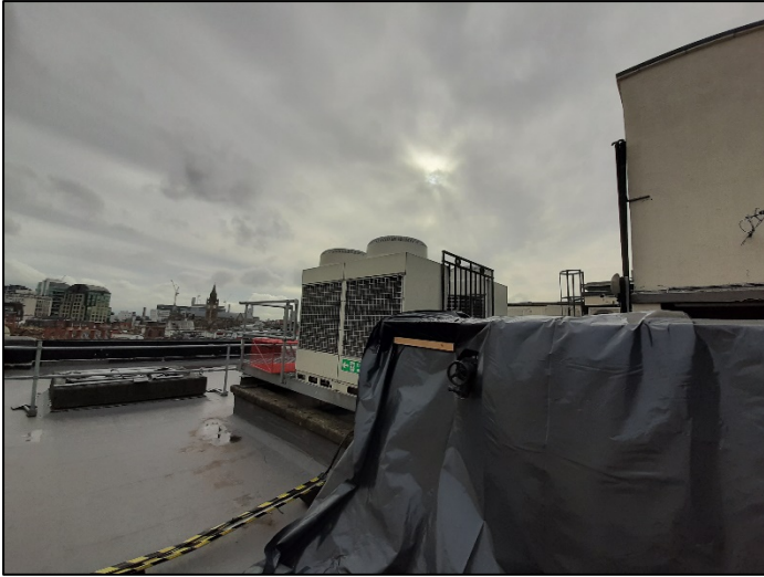
Photograph 8 –general roof ancillary structures
