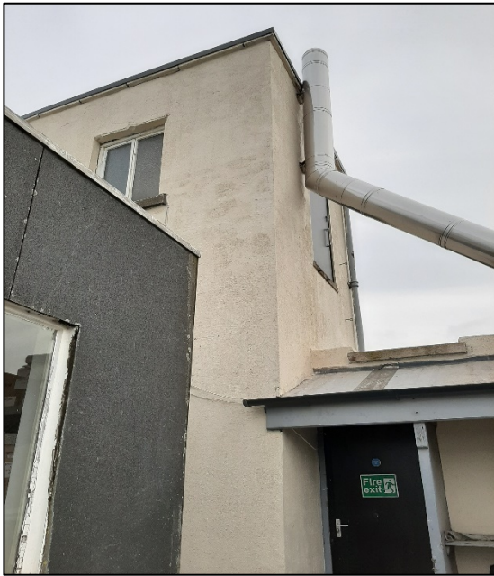
Photograph 6 – service lift building
