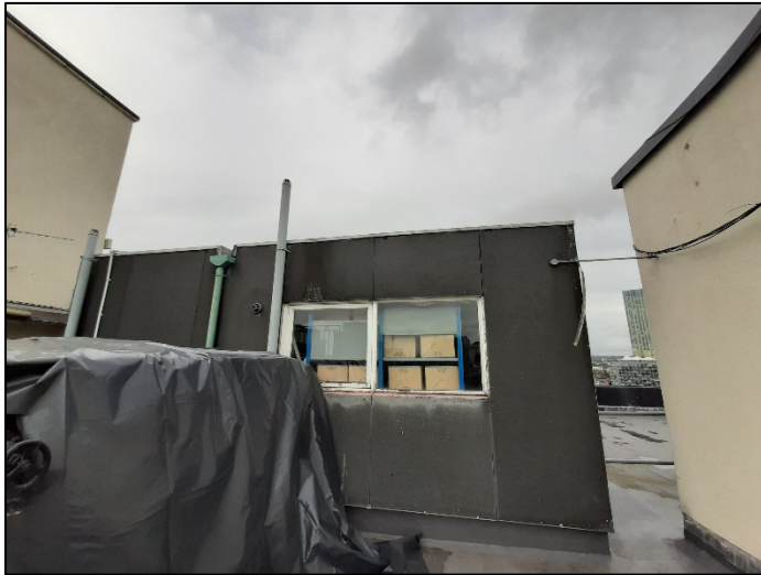
Photograph 4 – structure to be demolished
