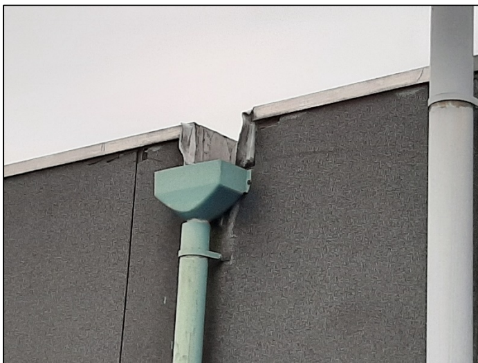
Photograph 5 – roofline on building to be demolished
