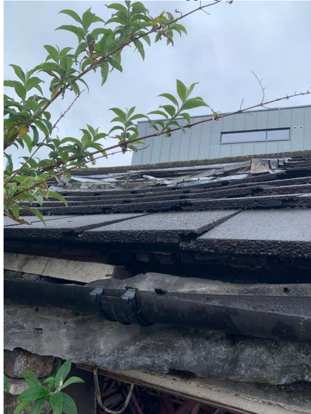
Roof Pitch 'sagging'
