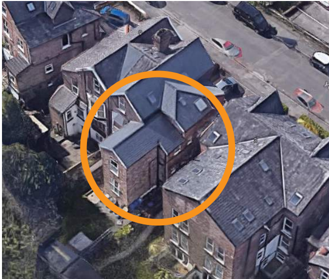
Two storey rear/side and roof extensions 7 York Road (108263_FO_2015_S1)
