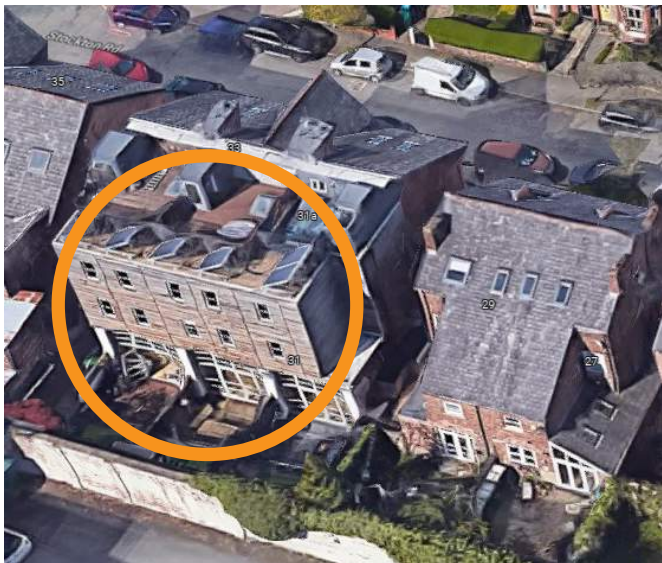
Timber clad rear extension and roof terraces 31-33 Stockton Road (081438_FO_2006_S1)
