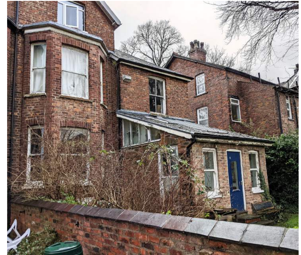
Top left: Frontages of No.s 1-5 Vincent Avenue Bottom left: Rear of No's.7-13 Vincent Avenue, viewed from the garden of No.5, showing existing rendered elevations Top right: Vincent Avenue from Oswald Road Bottom right: Rear of No.3 Vincent Avenue, viewed from the garden of No.5
