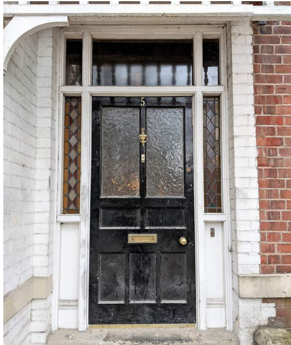
Original front entrance door and leaded stained glass side lights
