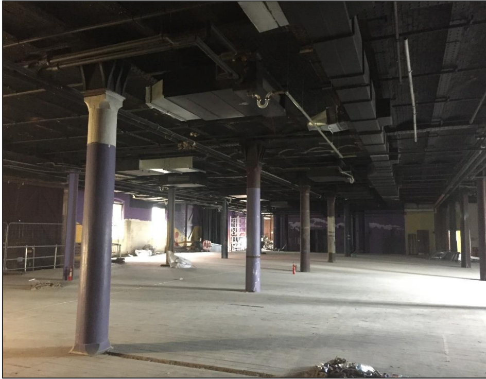
Figure 2: Level 3 of Grade II Listed Bonded Warehouse. Looking west across the space corner. March 2019. (SLHA).
