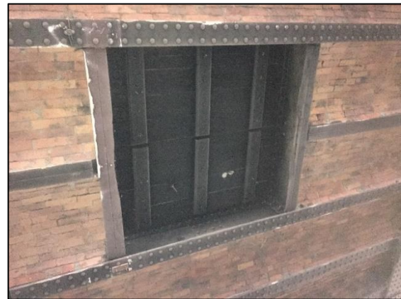
Figure 11: Original timber hatch to ceiling of Level 3. Site Visit, March 2019.
