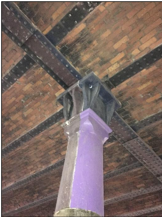
Figure 8: Circular section column and capital to Level 3. Site Visit, March 2019.
