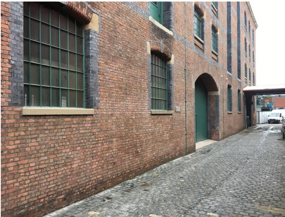
Figure 12: Bonded Warehouse, South Elevation. Example of original window / timber door. Note, the removal of the railway track. Site Visit, March 2019.
