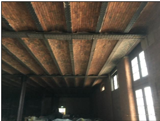
Figure 10: Typical ceiling arrangement at Level 3. Note the strengthening thickening plates added to the centre of the wrought iron beams. Site Visit, March 2019.
