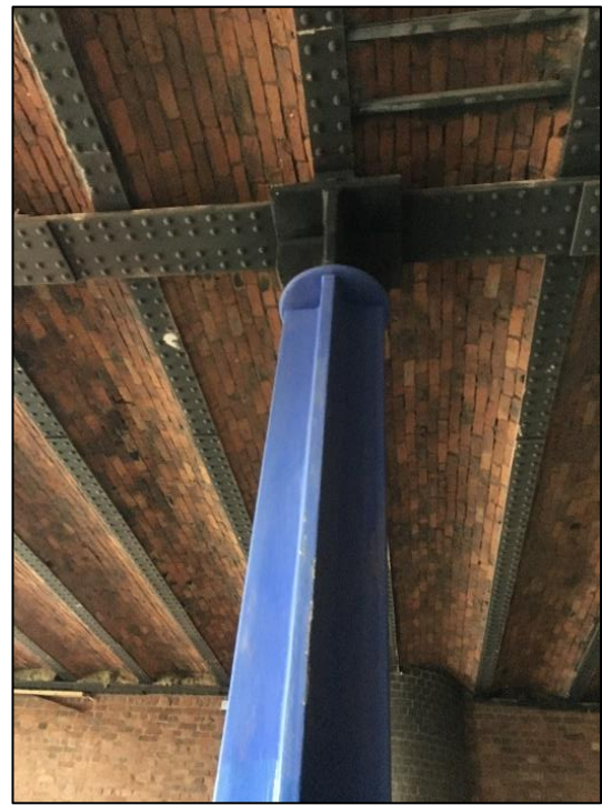
Figure 9: Slim cross section column and capital to Level 3. Site Visit, March 2019.
