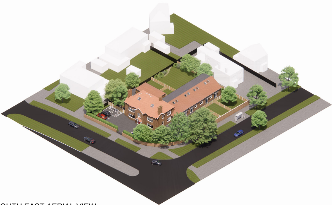
SOUTH EAST AERIAL VIEW
