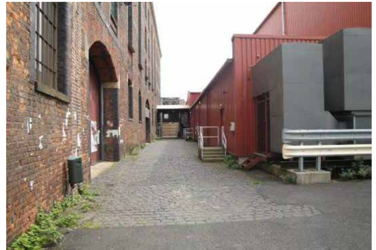
View of south elevation
