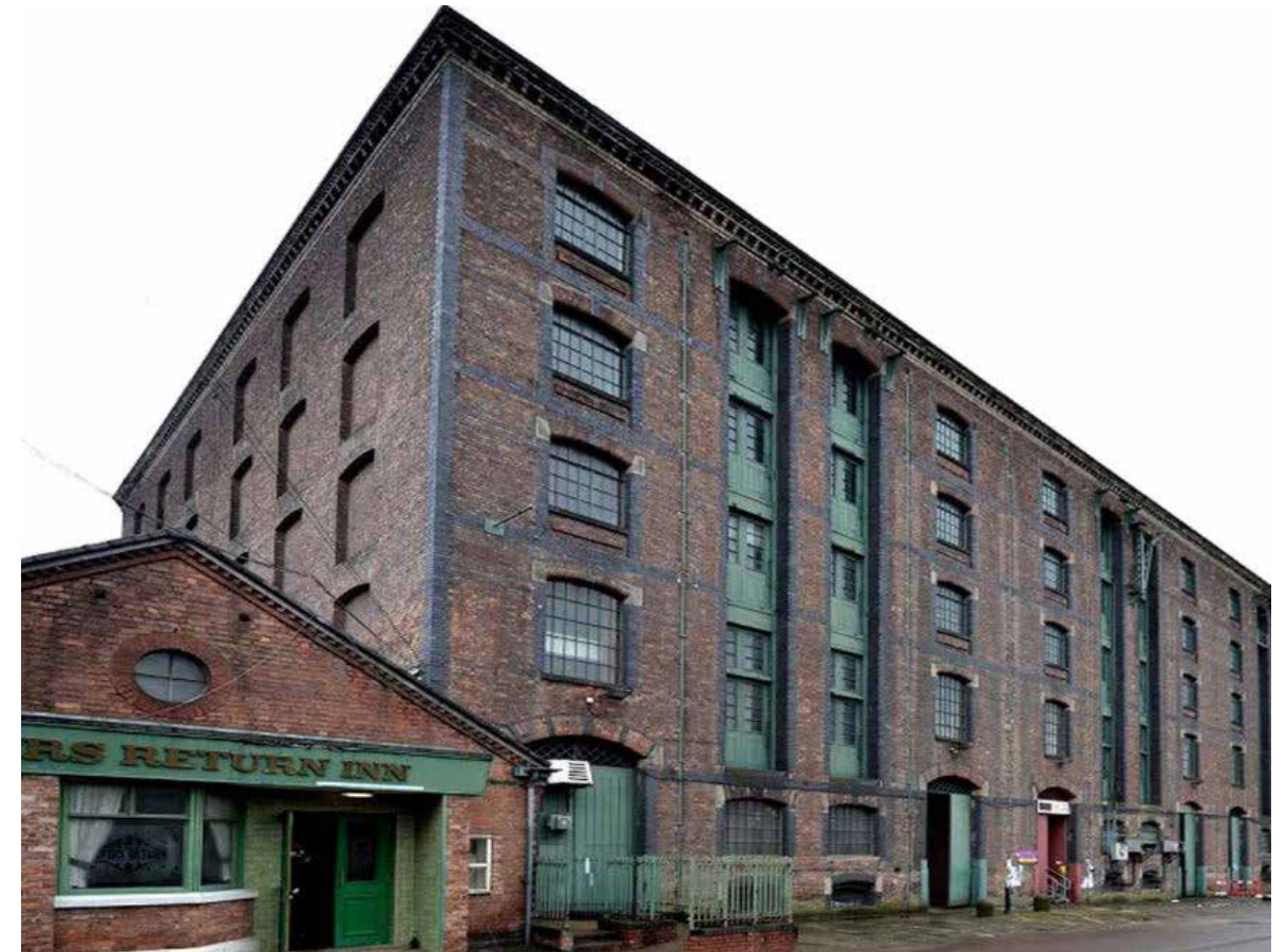
View of North East corner
