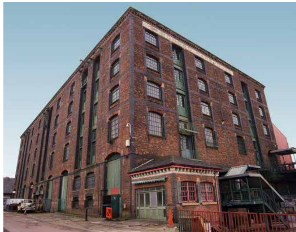
View of north west corner
