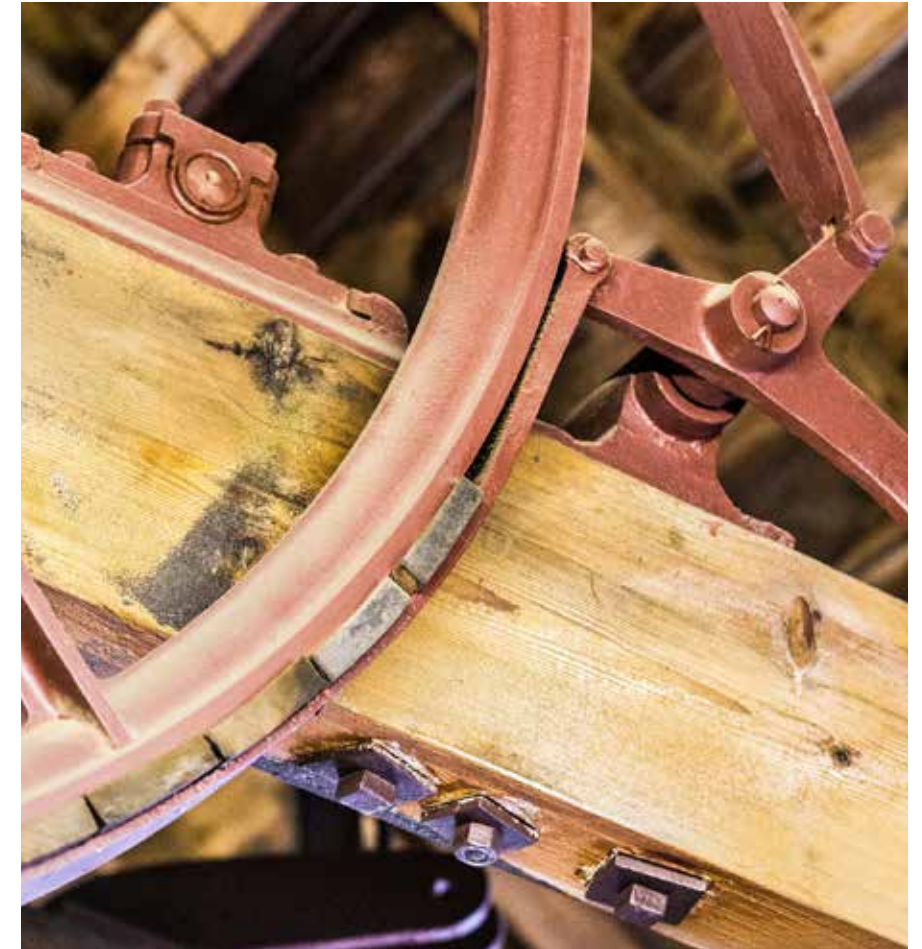
The sixth floor loft area boasts some original hoists and machinery.
