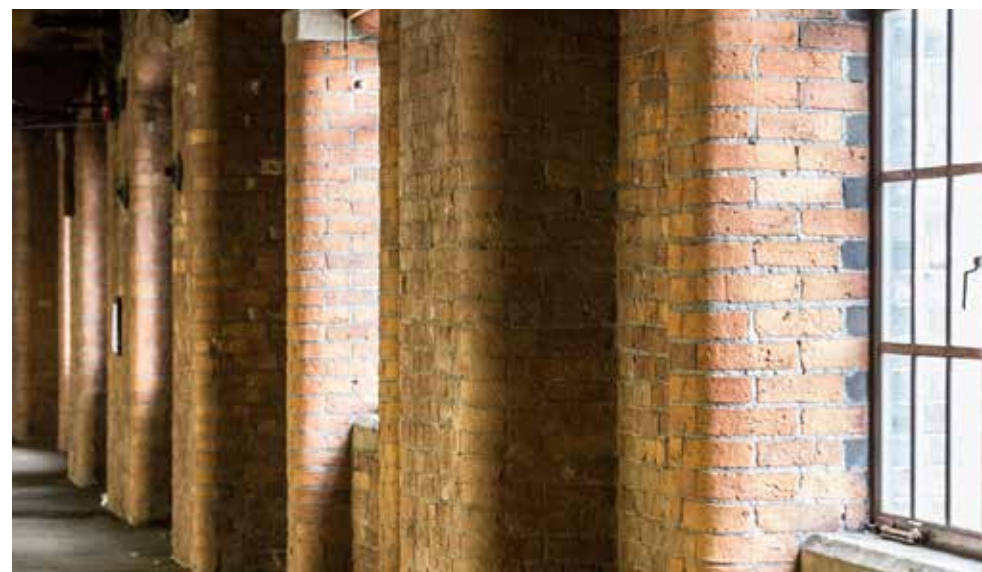
Typically the interior finish of the exterior walls are exposed brick
