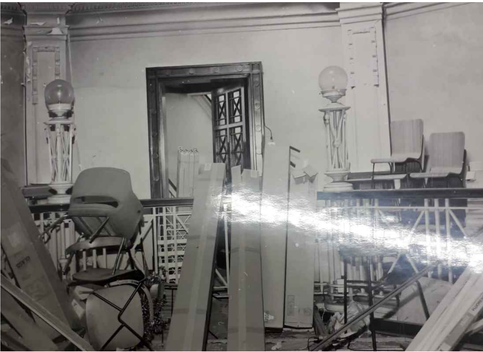
Photograph No. 05 Gallery Balustrading Detail (c. 1984)
