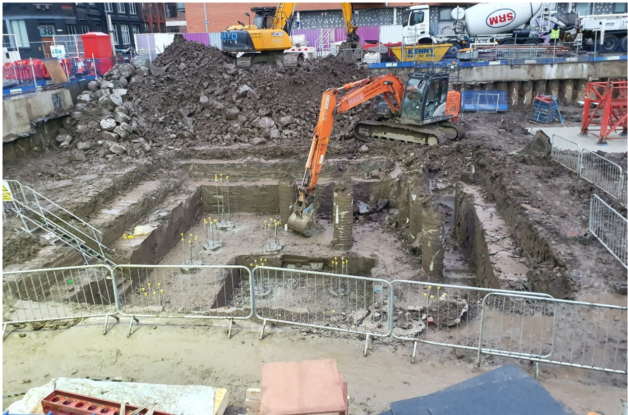
Photograph 1 – Basement excavation showing that all Made Ground soils have been removed.
