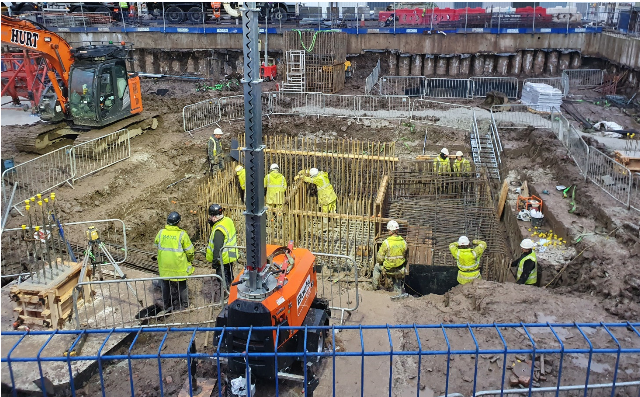
Photograph 2 – Basement excavation showing that all Made Ground soils have been removed.
