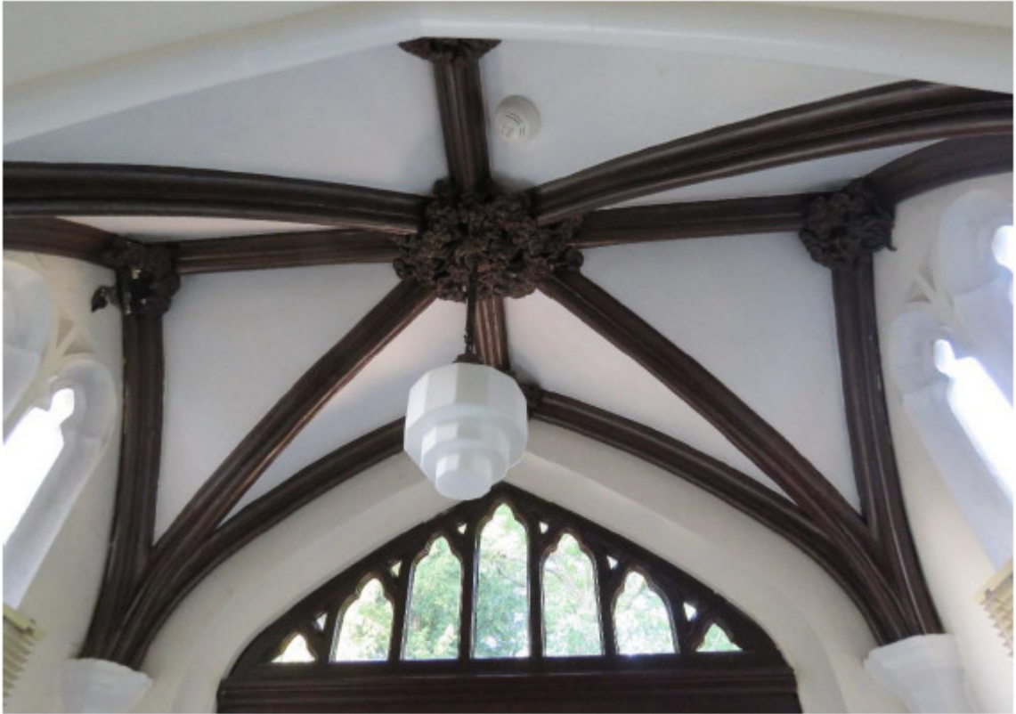
Fig 3.11 - Shows internal feature of the original vaulted ceiling.
