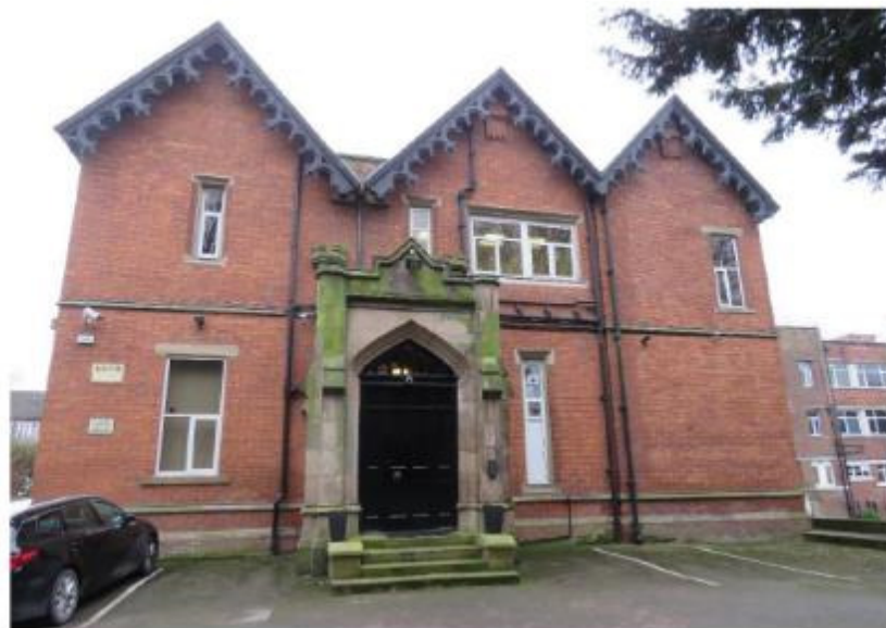
Fig 3.6 - Shows the north facing elevation retaining the original c1837 Gothic entrance porch, decorative bargeboards and stone detailing. Original windows have been removed.
