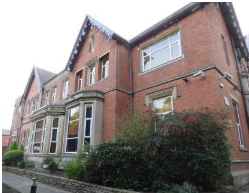
Fig 3.8 - Shows the east facing elevation with original decorative bargeboards, stone hoodmould windows and stone bays. It retains its original roofline and form despite the extensions. Original windows have been removed.
