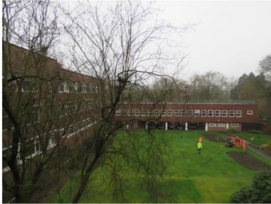
Fig 3.9 - View from the rear of the main house looking towards Platt Field Park, showing the open landscaped area to the rear. The low level extension allows long views of the parkland setting and tree line beyond, providing an association with the historic landscaped context.
