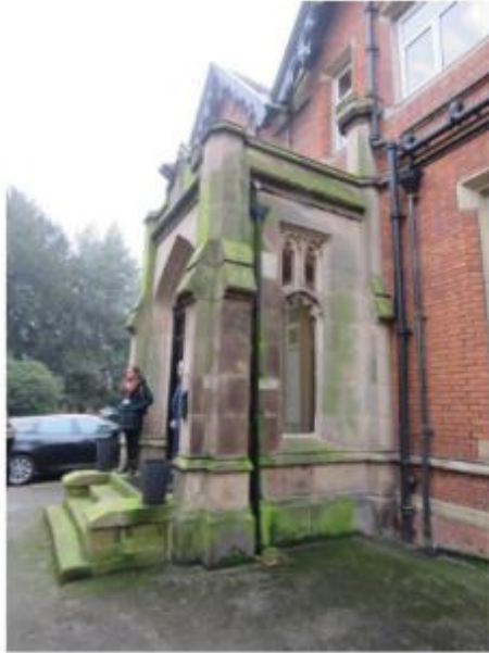
Fig 3.7 - Shows the Original grand Gothic porch with decorative stone tracery and castellated piers.
