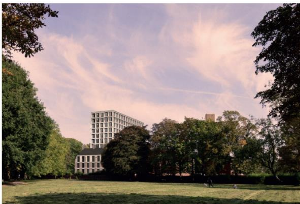
View to the west elevation of the scheme across Platt Fields Park
