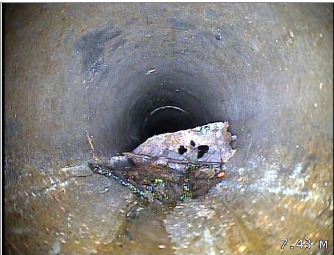
Other settled deposits 5% cross-sectional area loss - Remark: LEAF
