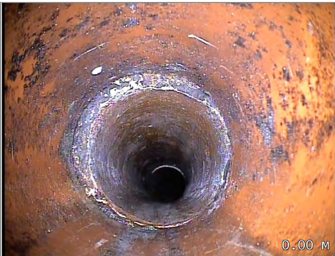
Start node type, manhole, reference MH 01
