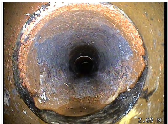
Attached deposits, encrustation from 3 to 8 o'clock 5% cross-sectional area loss
