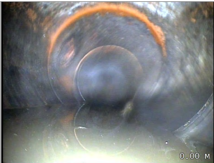
Start node type, manhole, reference MH 03
