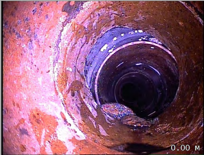
Start node type, manhole, reference MH 02
