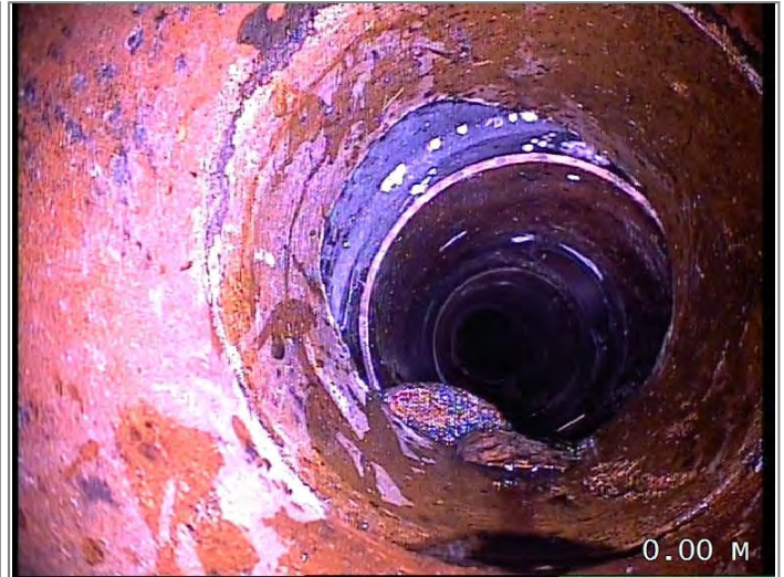
Water level 5% height/diameter
