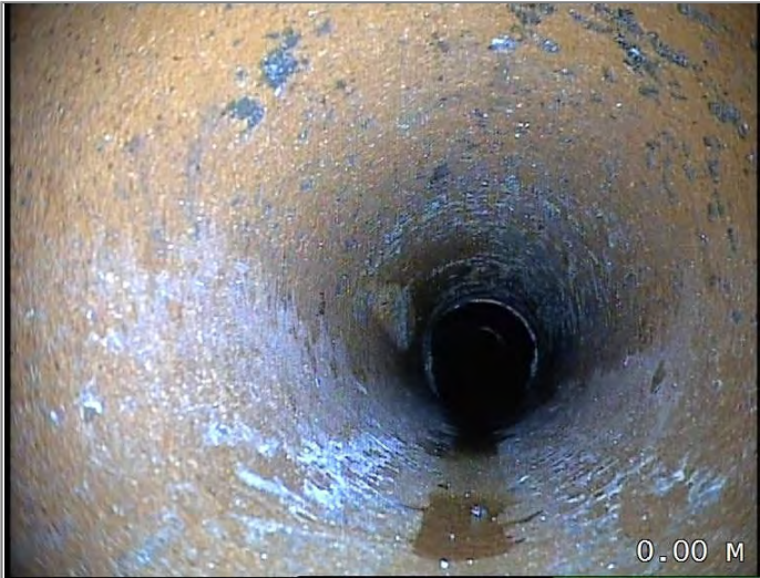
Start node type, manhole, reference MH 02
