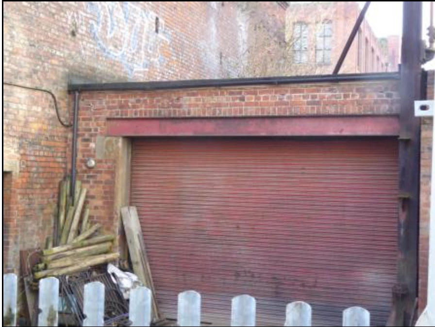
Photograph 10 showing the exterior of the garage attached to the Engine Room
