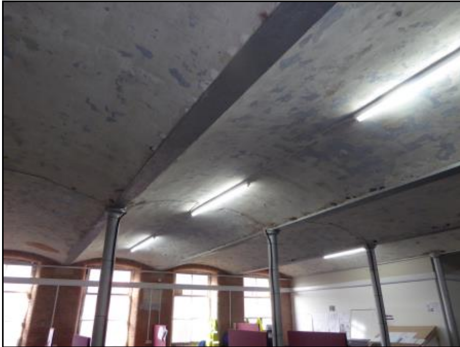
Photograph 5 showing the interior vaulted ceiling of one of the industrial units
