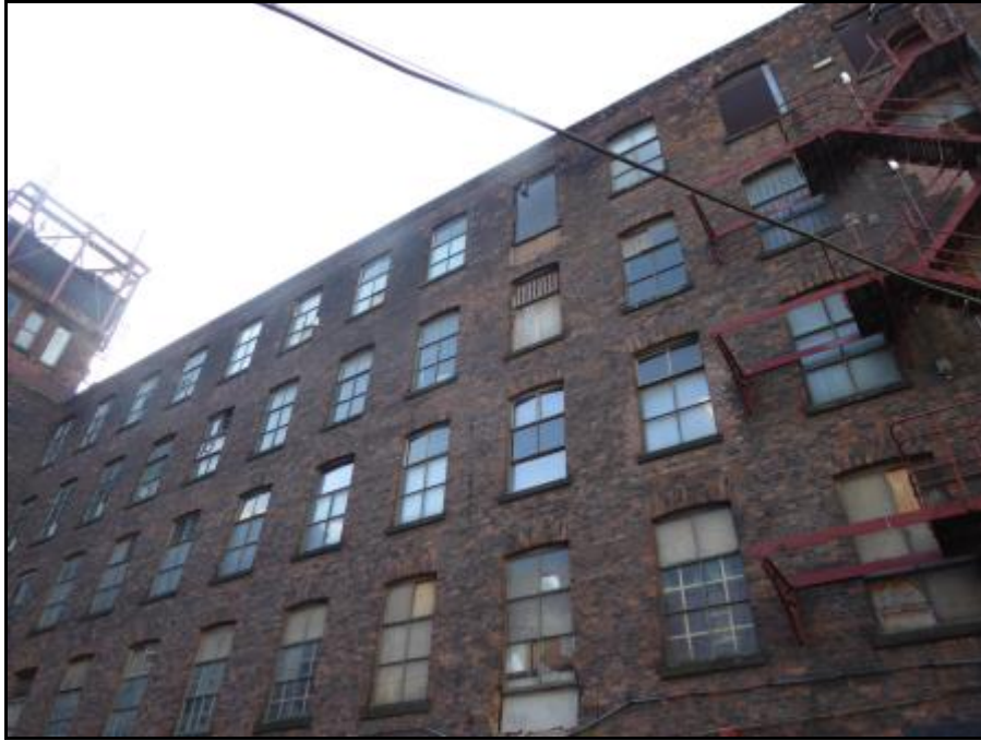
Photograph 1 showing the brickwork at the front elevation
