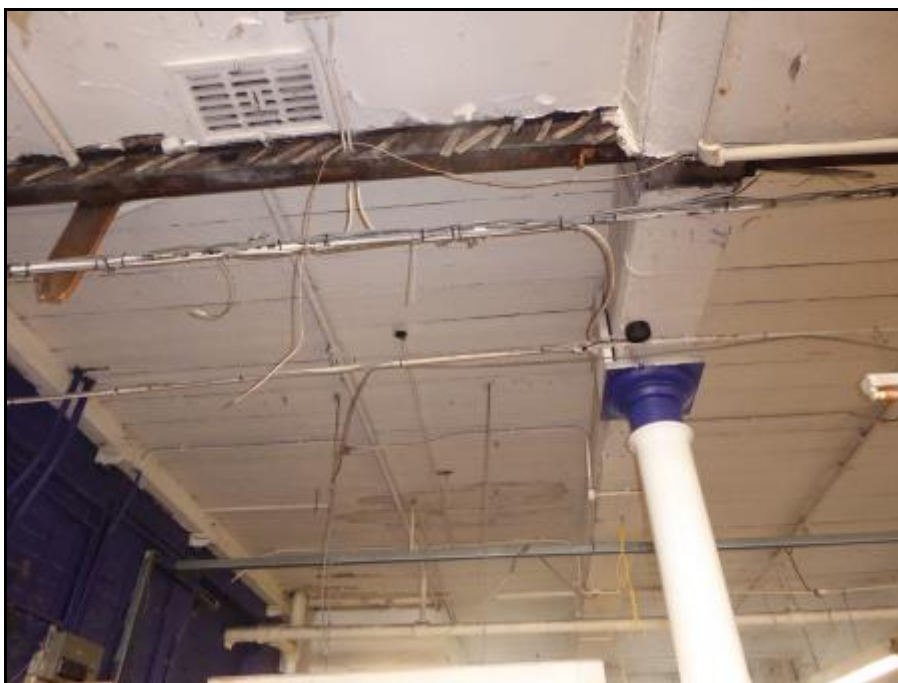
Photograph 6 showing a panelled ceiling
