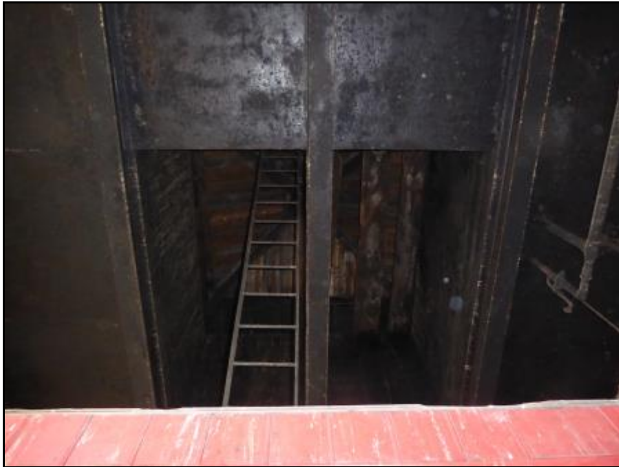
Photograph 7 showing the wooden timbers of the tower
