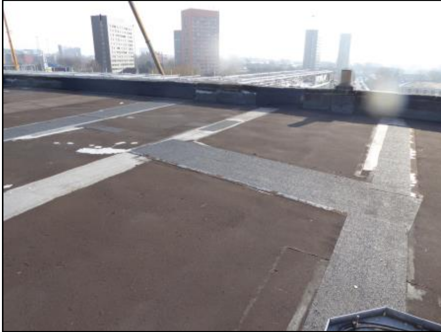
Photograph 3 showing the flat roof of the property
