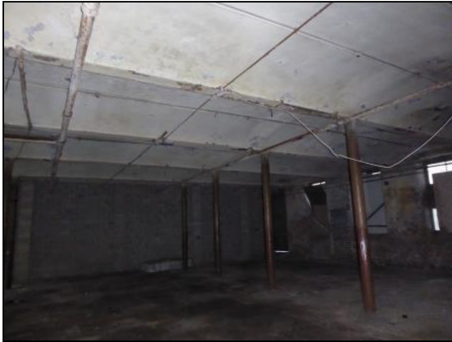
Photograph 8 showing one of the basement sections
