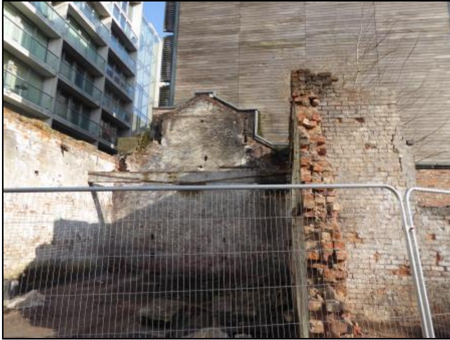
Photograph 14 showing the remaining brick walls of Building C
