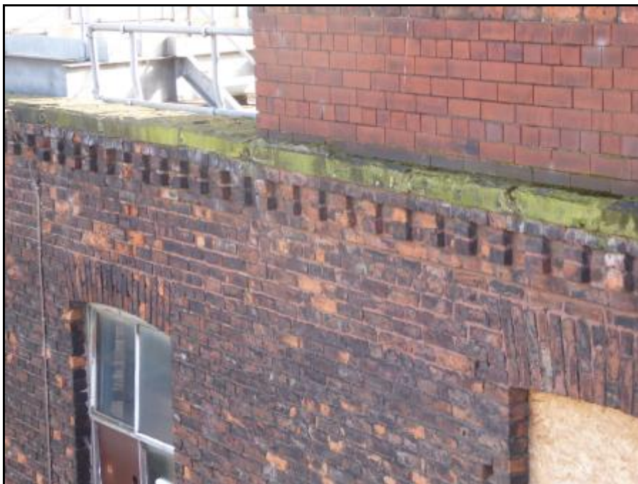
Photograph 4 showing the roof edges
