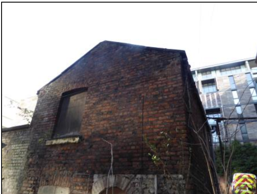
Photograph 12 showing the exterior brickwork of Building D
