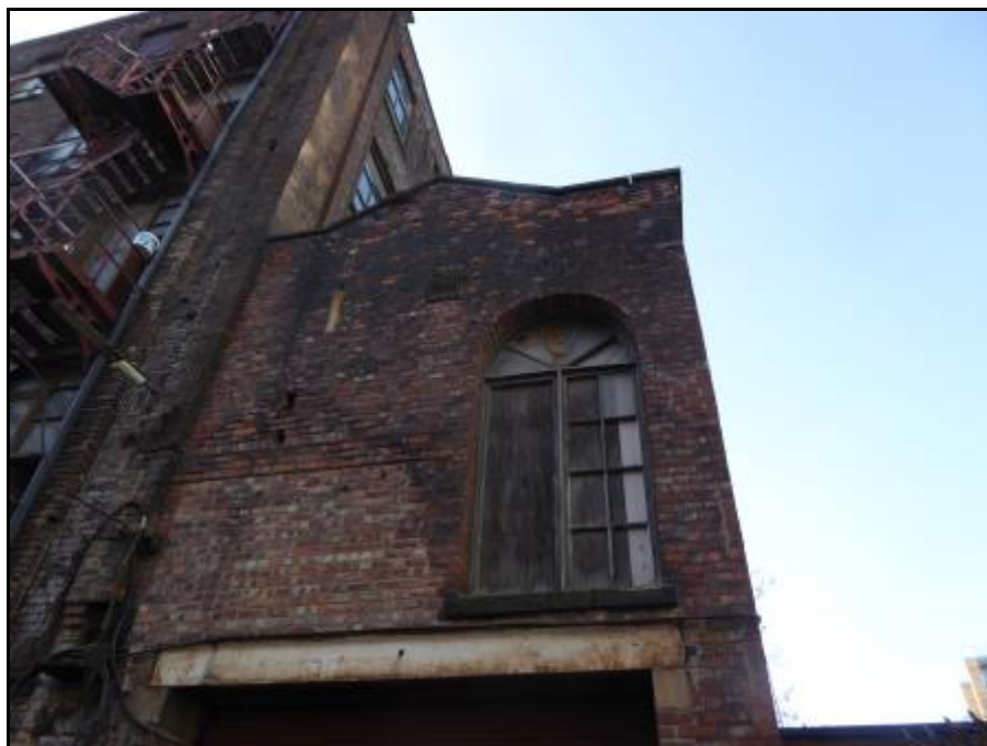
Photograph 9 showing the exterior of Building A (Engine House)
