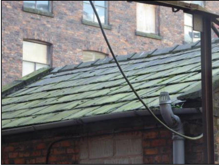
Photograph 13 showing the roof of the Building D
