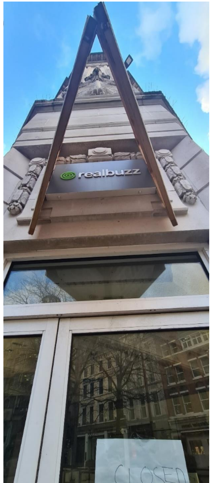
Stonework Detail above doorway
