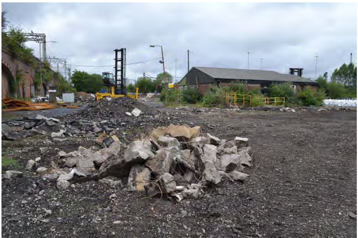
Plate 32: Sightline to the north-west along the Site's western boundary.
