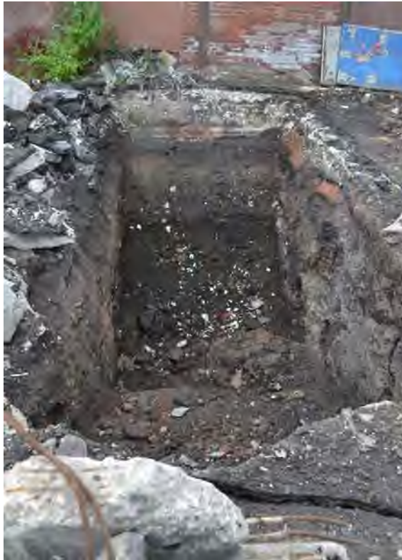
Plate 27: Recently excavated trial pit adjacent to the railway viaduct. The absence of structural remains is not surprising as this location does not correspond with any known structure shown on the historic mapping, but it does highlight the depth of the Made Ground.
