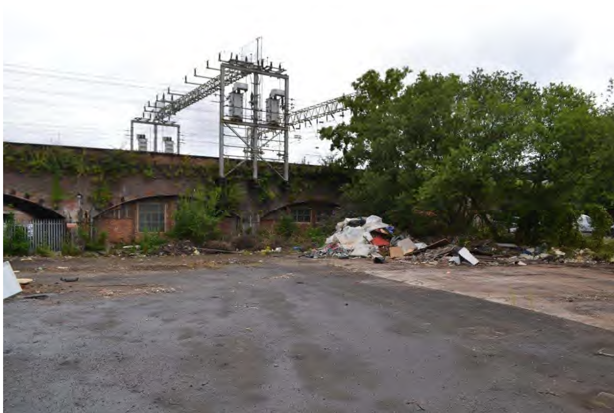
Plate 20: Sightline to the Site's north-western corner showing the intersection of the Site's northern boundary with the railway viaduct.
