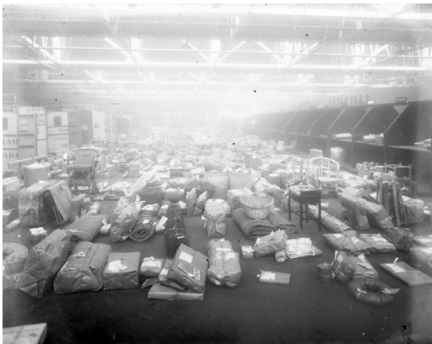
Photograph. Interior view of Bennett Street Parcel Depot, 22 Feb. 1929 (City Engineers Department), Manchester Libraries, Information and Archives ref. GB127.m77482
