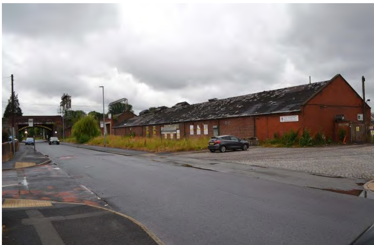
Plate 2: Sightline to the west along Bennett Street showing the former Parcel Depot building. The overgrown grass area in front of the building is the Site of the terraced housing (GMHER ref. 13853.1.0) which occupied that location from c. 1890s – c. 1980s.
