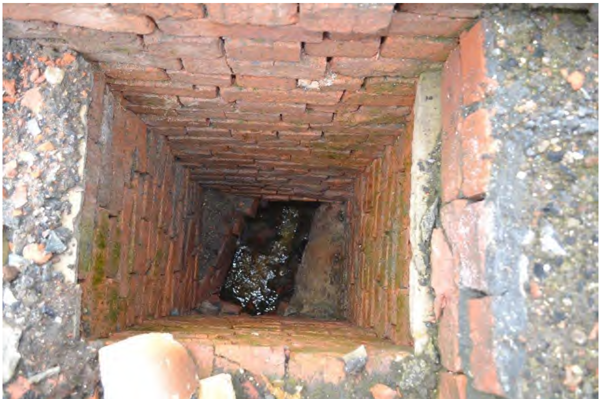
Plate 26: Sightline down the brick-lined access shaft to a culverted watercourse, probably the Corn Brook.
