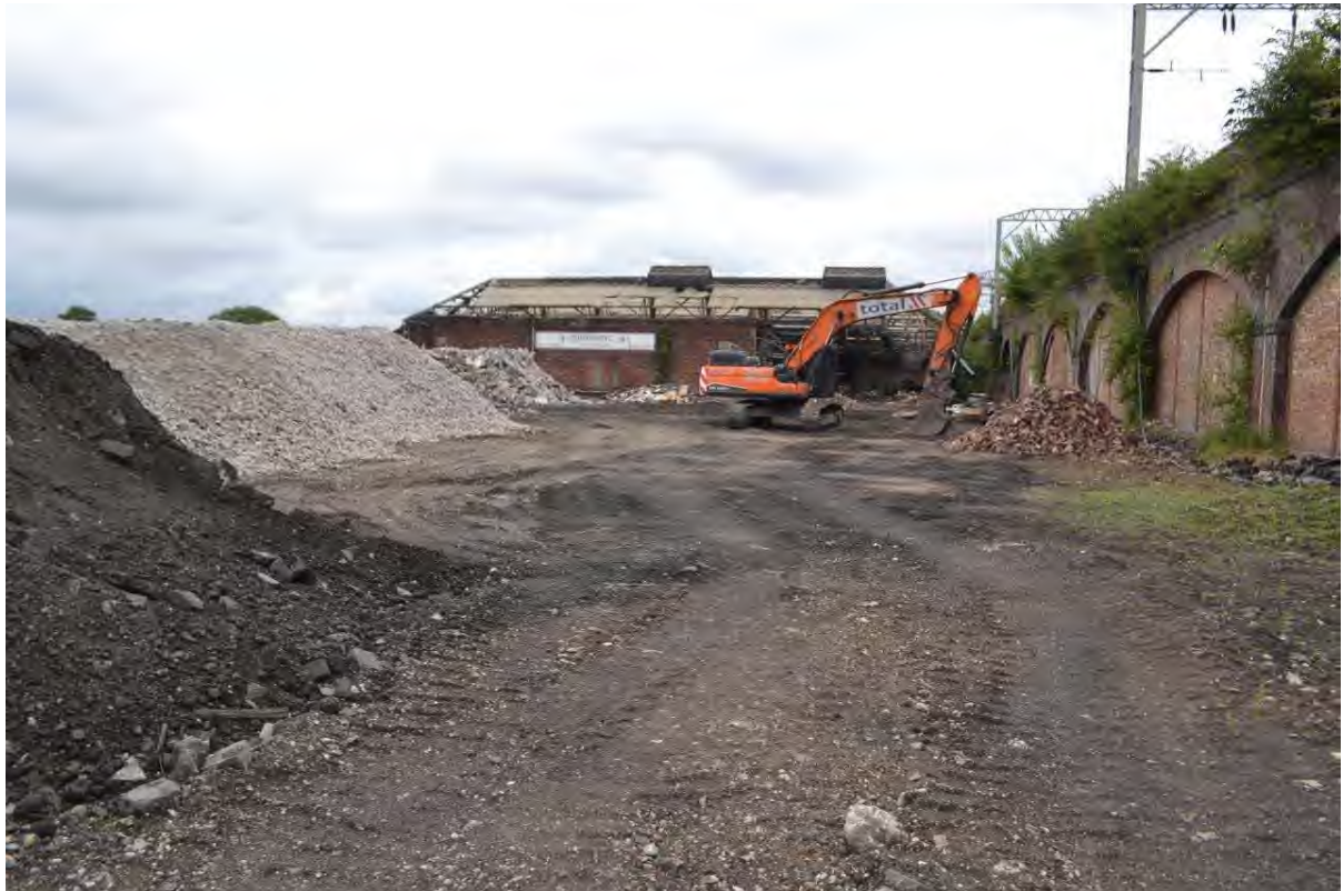
Plate 31: Sightline to the south-east along the Site's western boundary towards the north-western facing elevation of the former Parcel Depot.
