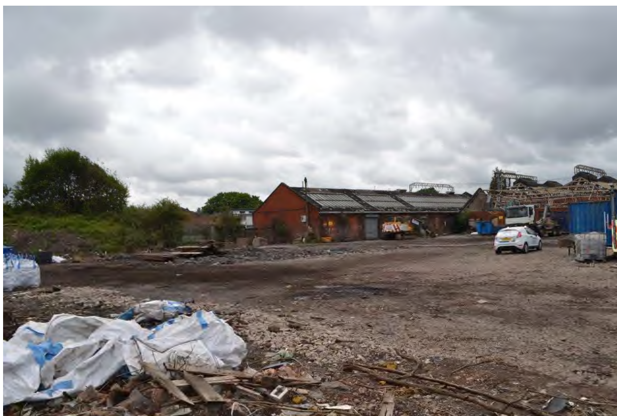
Plate 6: Sightline to the south-west towards the Site entrance and the former Parcel Depot building.
