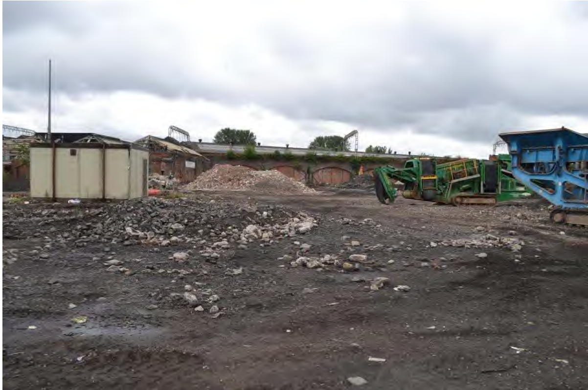
Plate 9: Sightline to the west across the centre of the Site towards the railway viaduct.
