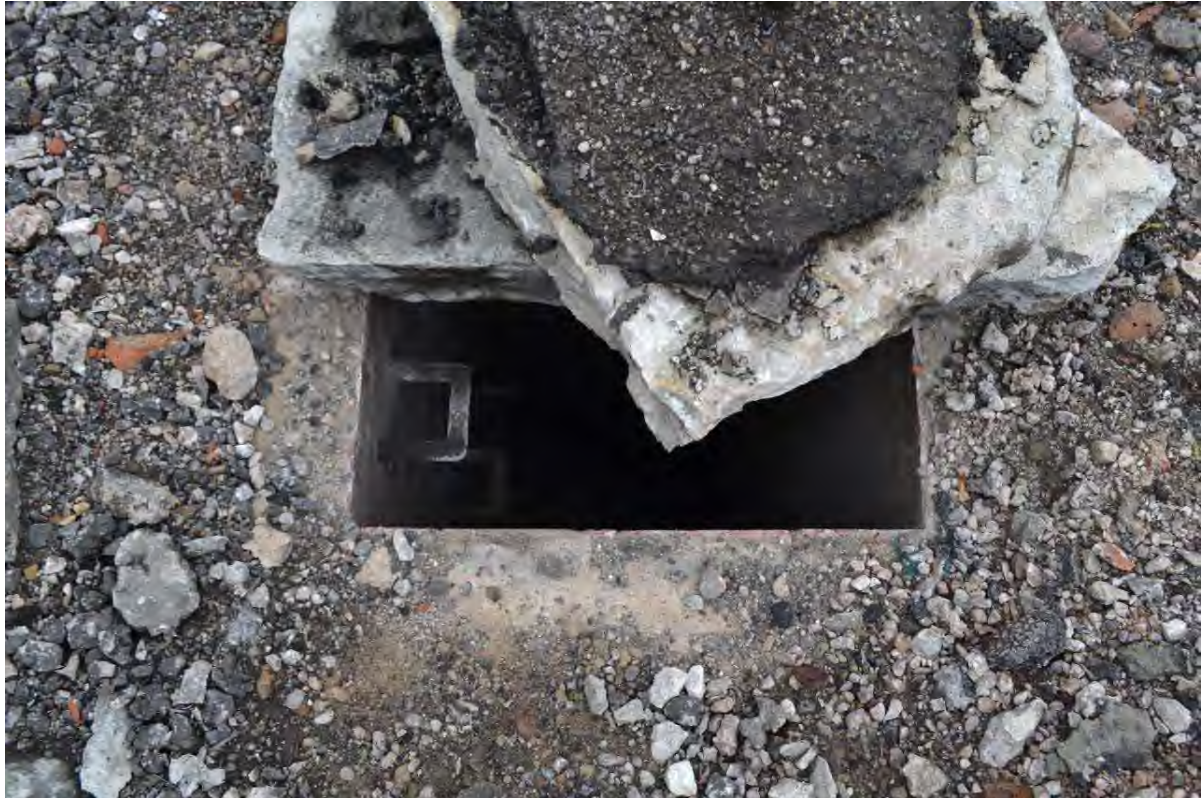
Plate 29: Brick-lined access shaft
