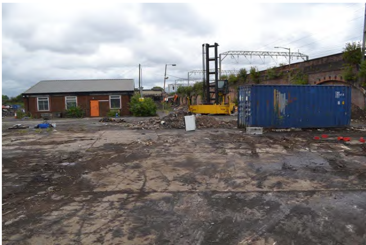
Plate 24: Sightline to the south-east along the Site's western boundary with the railway viaduct
