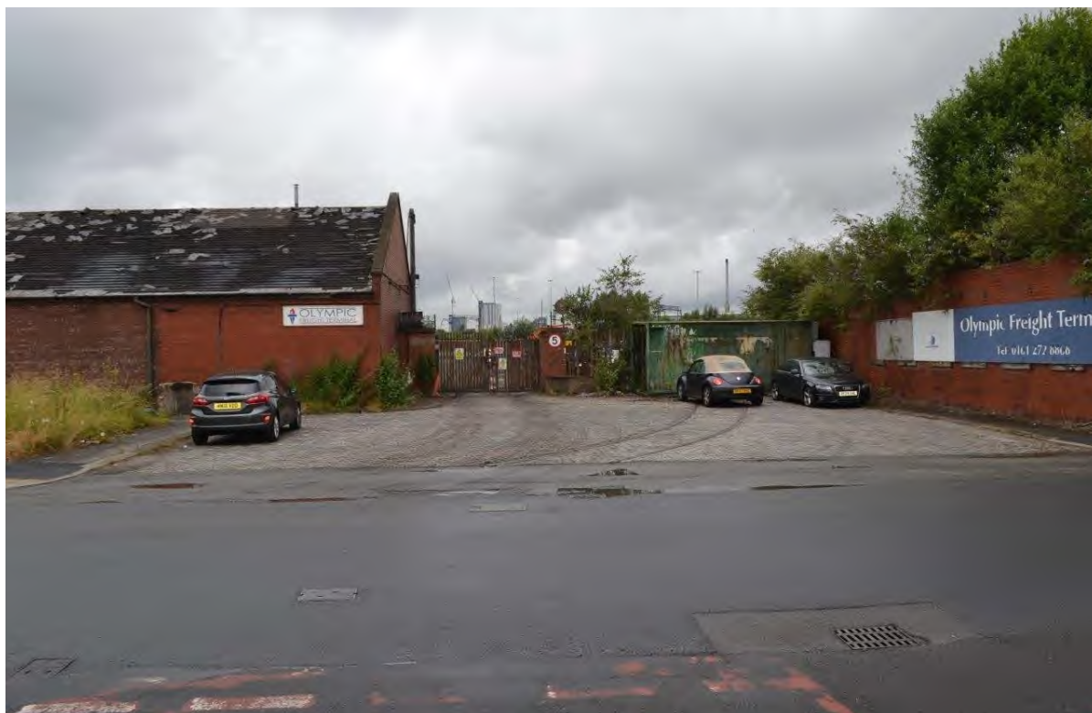
Plate 1: Sightline to the north-west from Bennett Street towards the Site access. The former Parcel Depot is to the left and the arcing parallel tramway tracks extending into the former Permanent Way Depot as shown on the OS map of 1935 (Fig. 12 above) are clearly visible leading to the black VW Beetle
