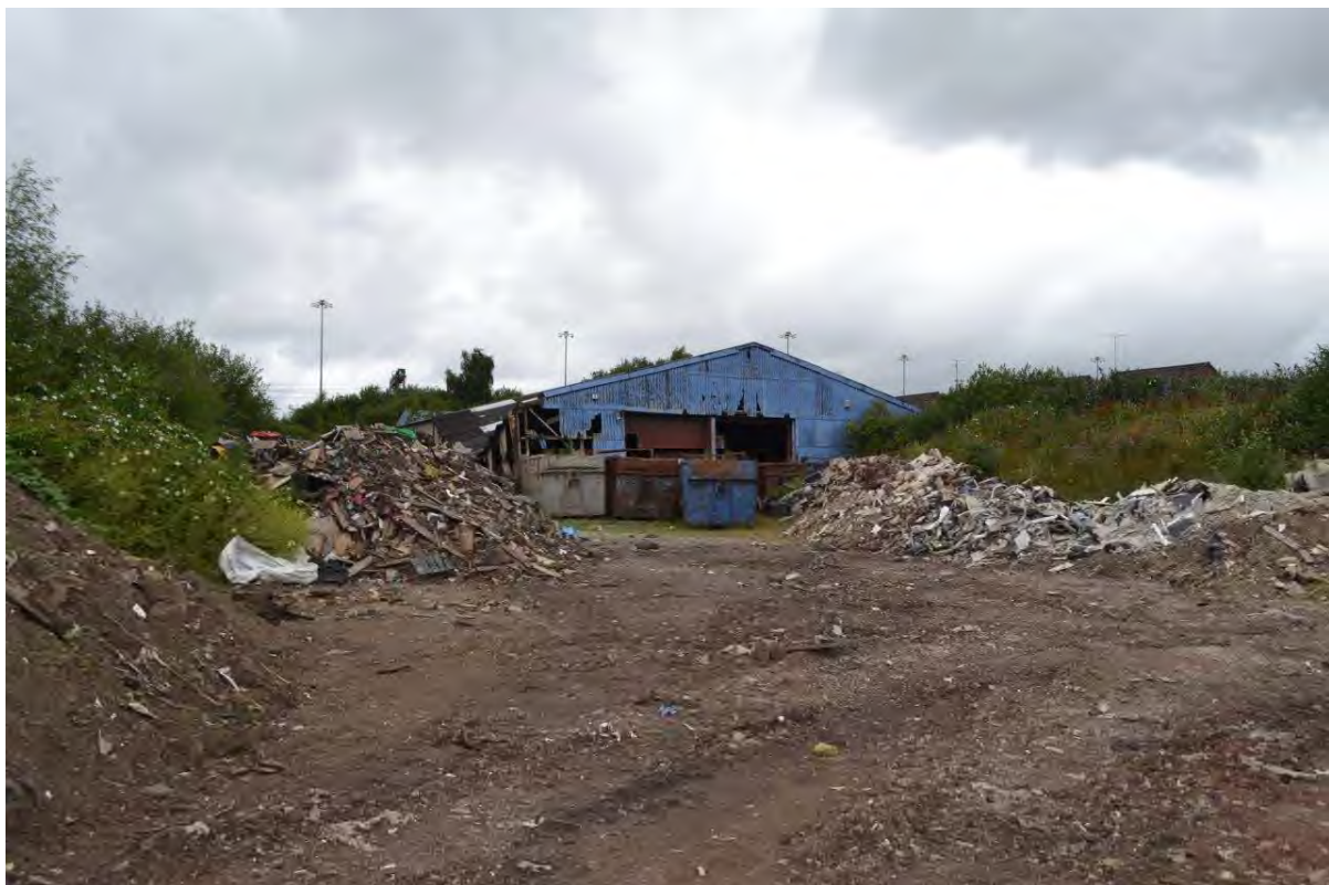
Plate 10: Sightline to a dilapidated building constructed in the late 1980s – early 1990s in the north-eastern corner of the Site.
