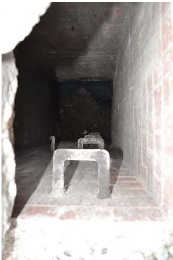
Plate 30: Sightline down the brick-lined access shaft to a culverted watercourse, probably the Black Brook
