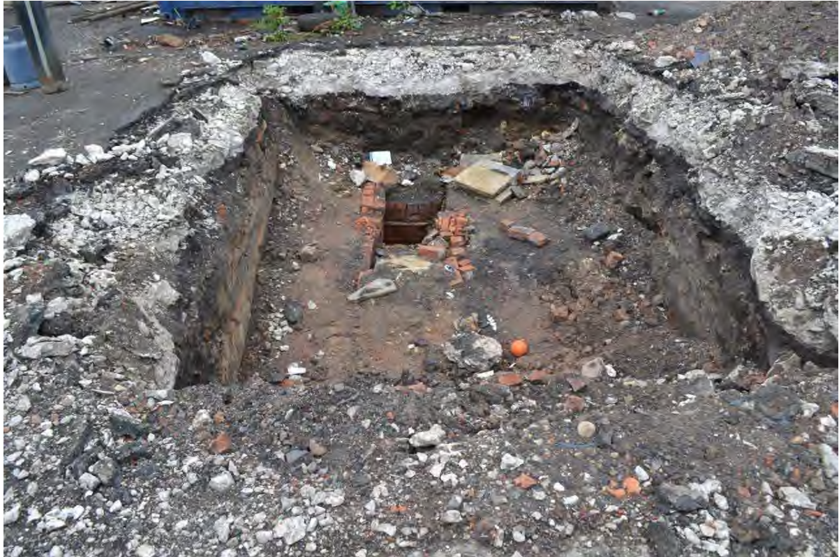
Plate 25: Recently excavated trial pit locating a brick-lined access shaft within the footprint of the Bennett's Iron Foundry (GMHER ref. 9683.1.0). Note absence of any other structural remains or floor surfaces.
