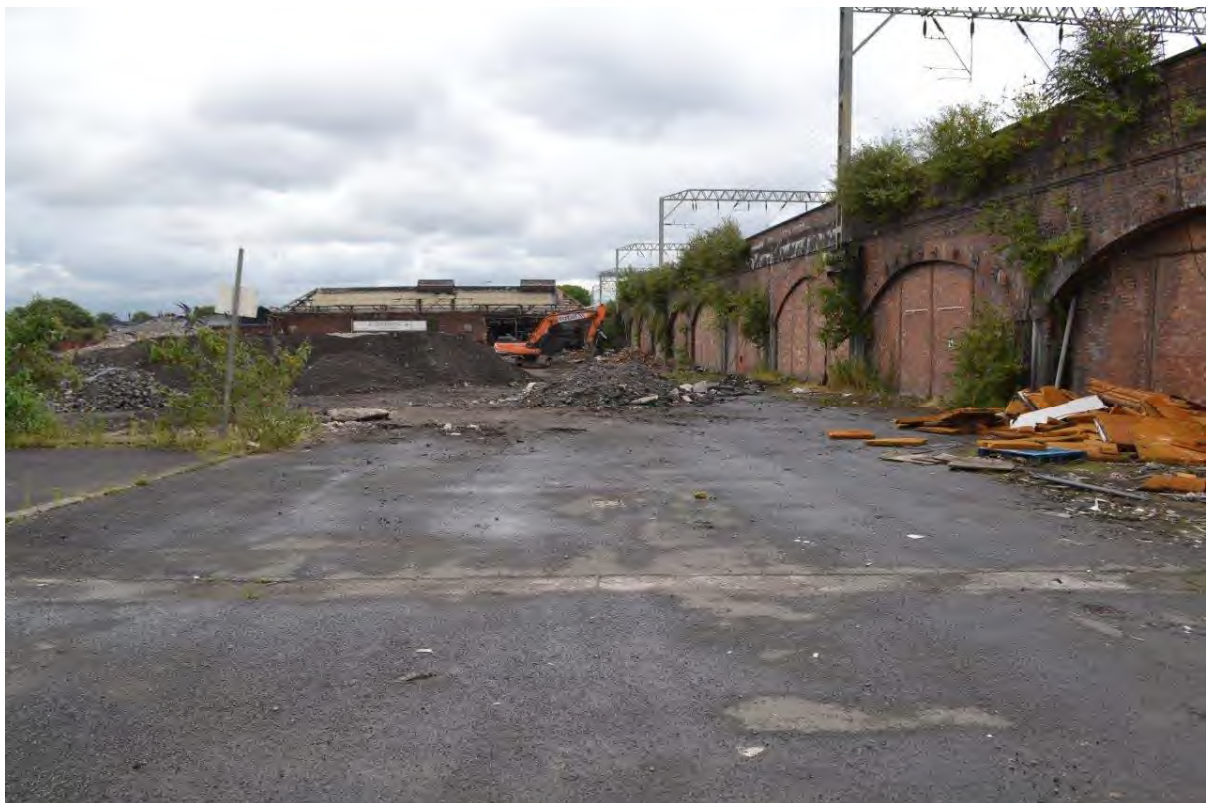
Plate 28: Sightline to the south-east along the Site's western boundary towards the north-western facing elevation of the former Parcel Depot.
