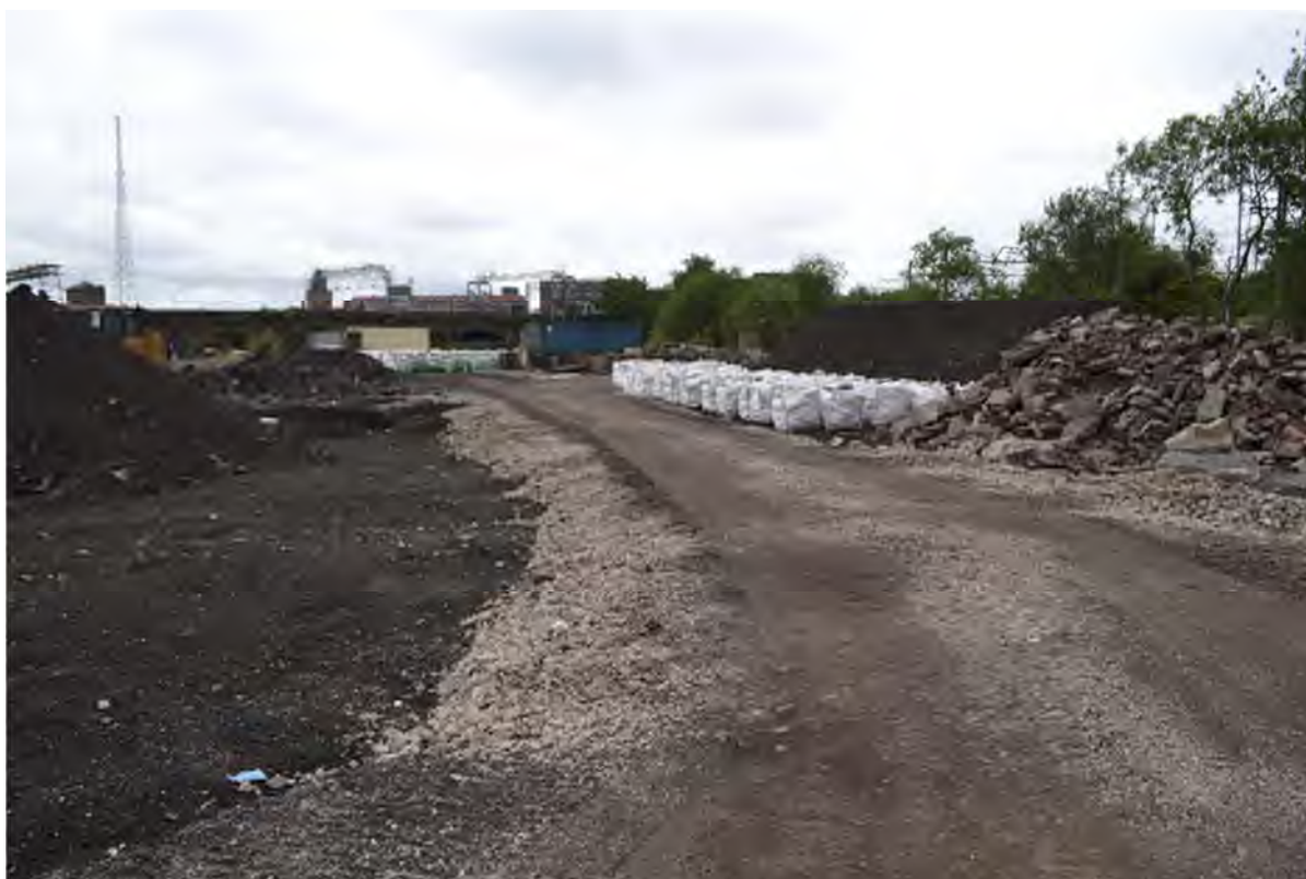
Plate 14: Sightline to the west along one of the temporary vehicle routes established using granular material.
