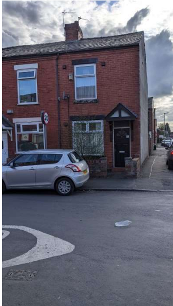
Front Elevation from Randolph Street.
