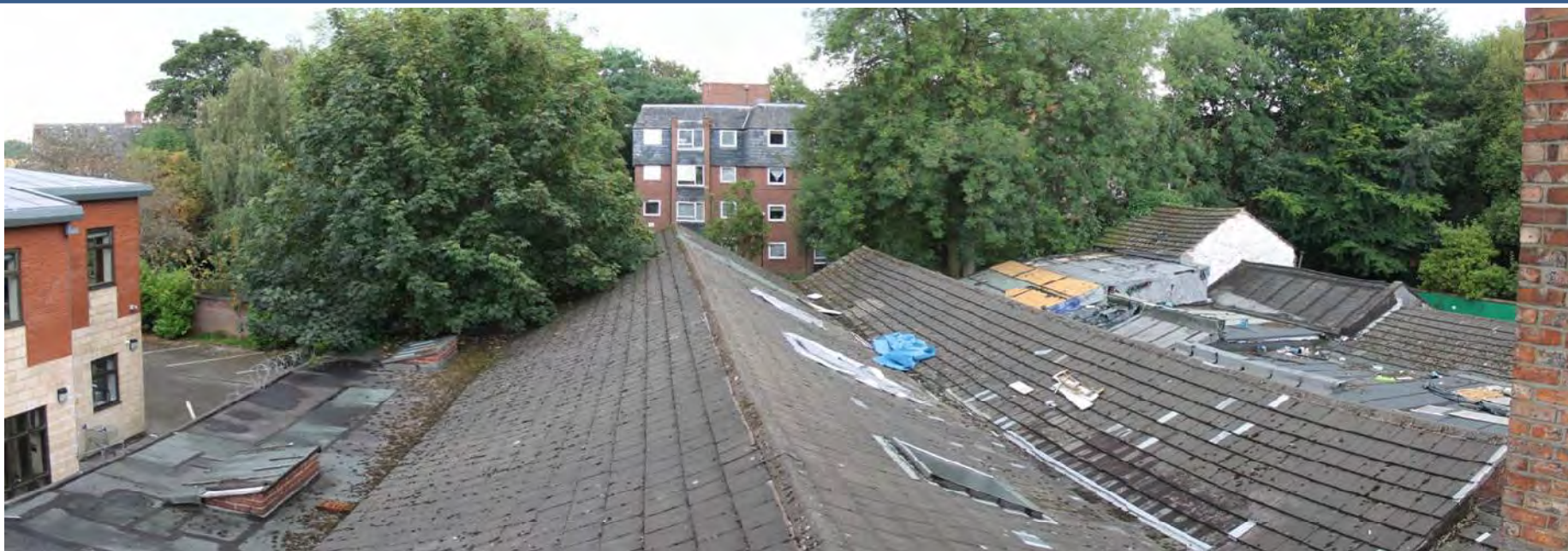
Photo 9: Taken from a first floor fire escape at the rear of the main building looking across the warehouse roofs
