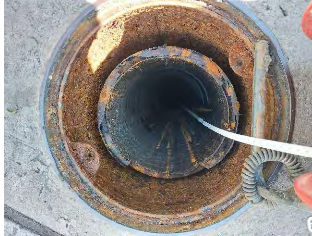
Image 8: 30 m deep UST monitoring well in the north near the tank farm.
