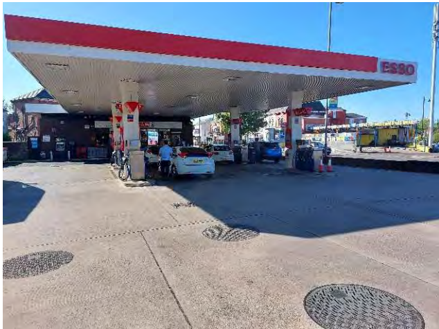
Image 1: View of forecourt from the northwest. Tank farm located here.
