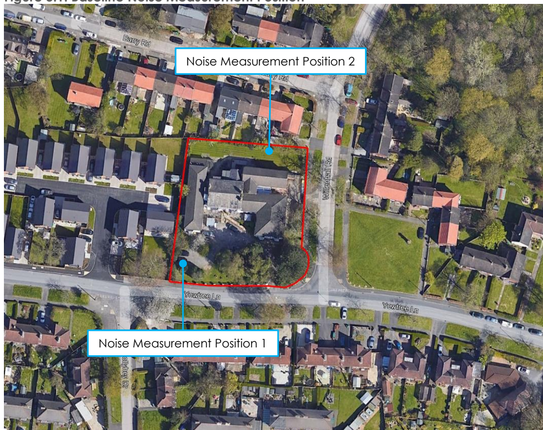
Figure 3.1: Baseline Noise Measurement Position
