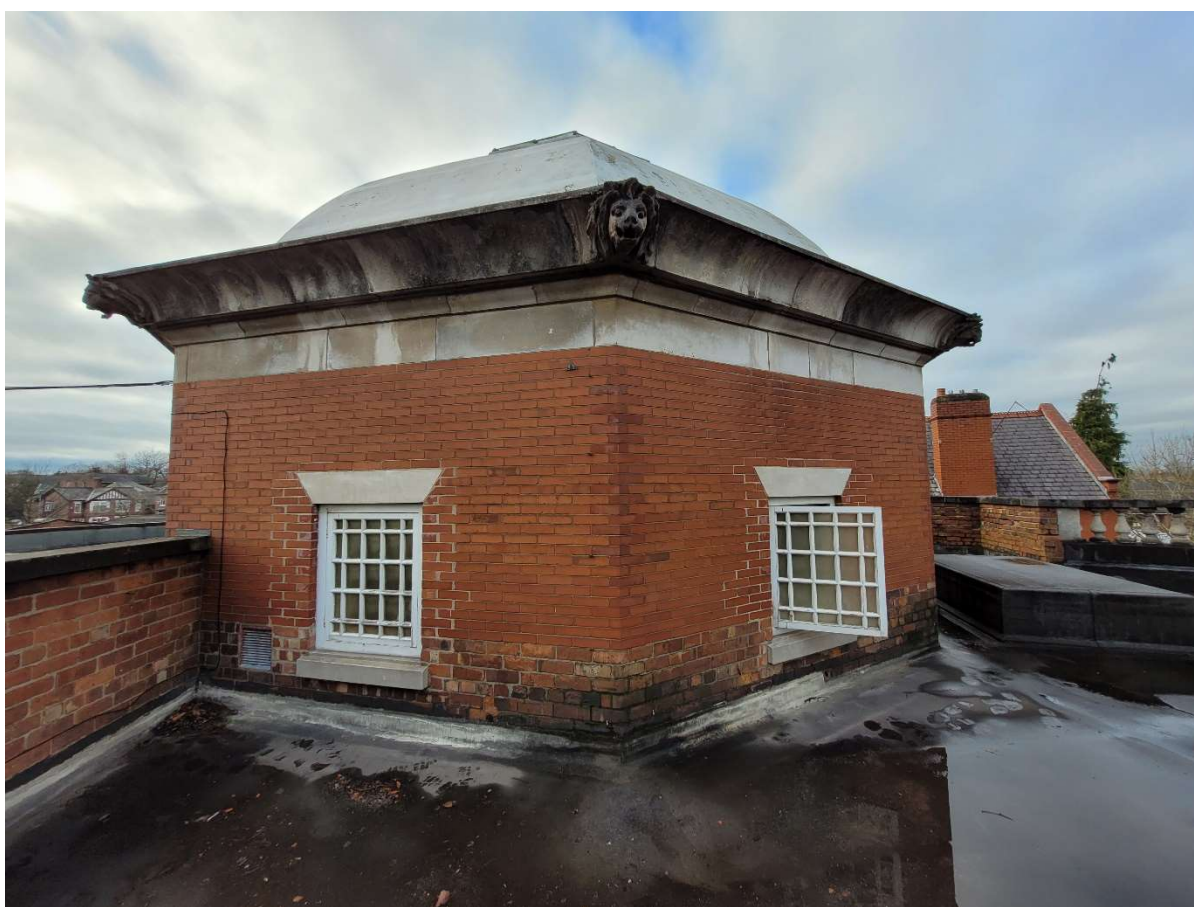
Rotunda and abutting asphalt roof from the east parapet.
