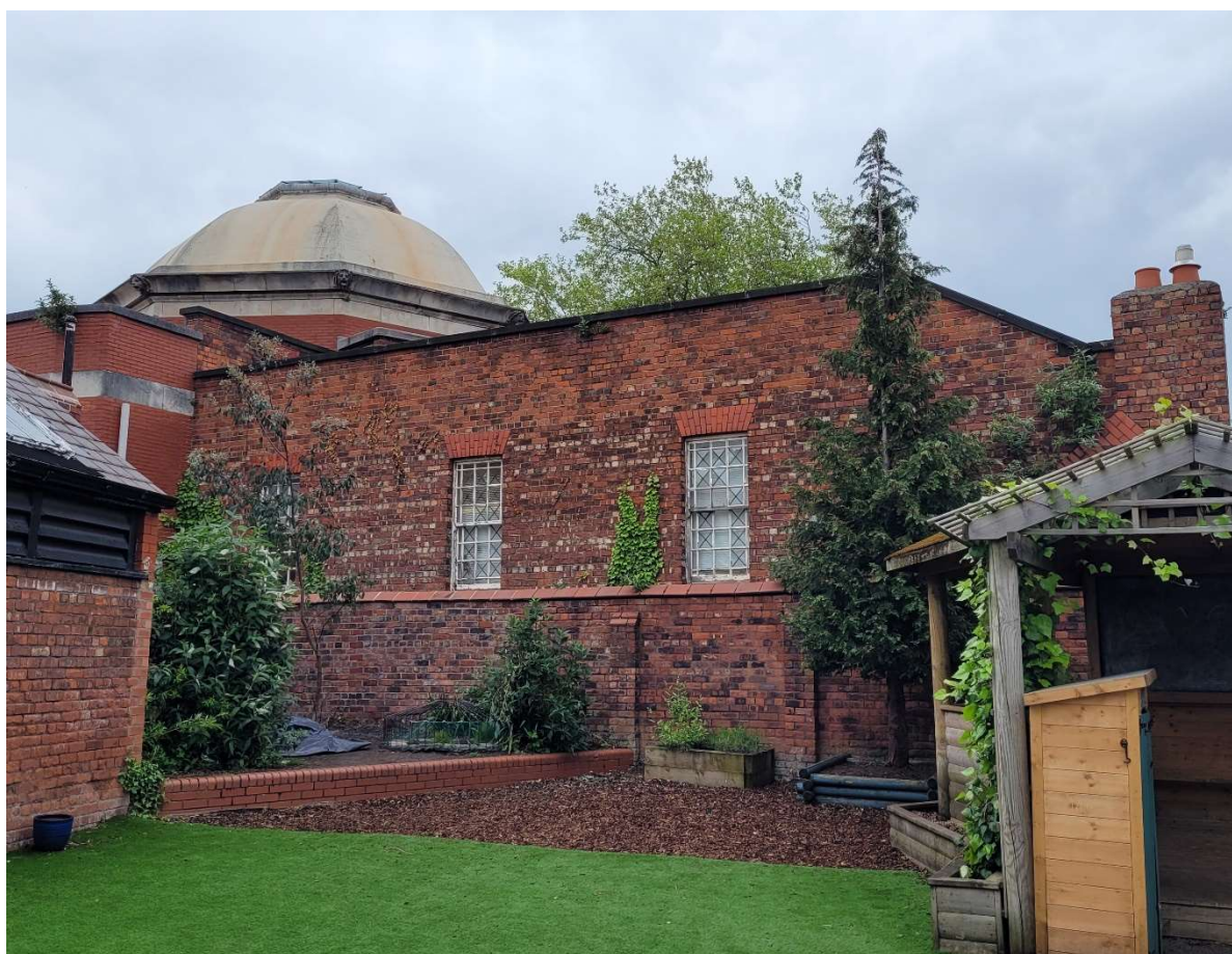
The north-west wall of the original building from the adjacent school.
