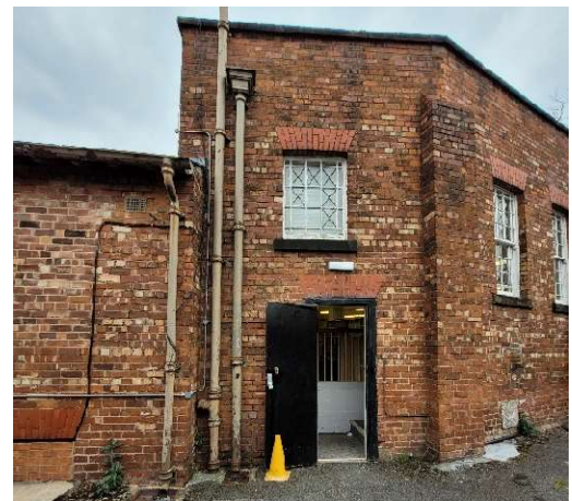
Extension abutment to the south/west walls of the original building. Store doors and roof to be renewed.
