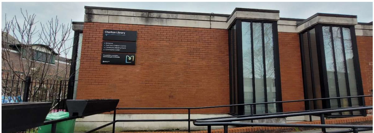
Extreme south end of the extension east wall facing Manchester Road.
