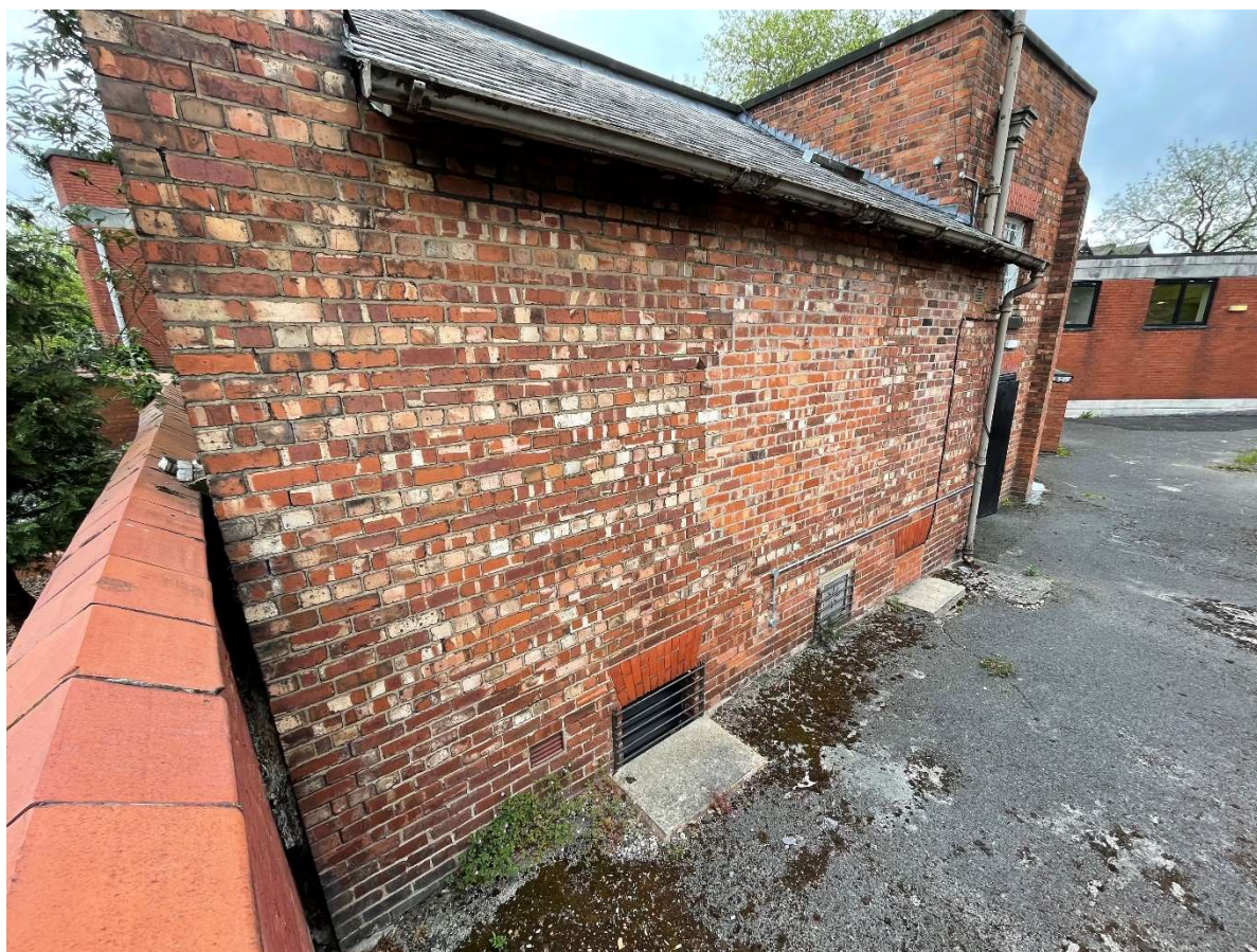
The much altered wall to the service yard beneath the slated roof, and over the basement boiler house.
