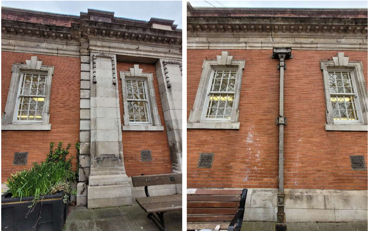
Details in the centre section of the east wall of the Listed Building.
