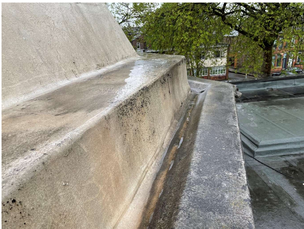
Asphalt finishes to Rotunda roof and parapet gutter, note corner gargoye outlet
