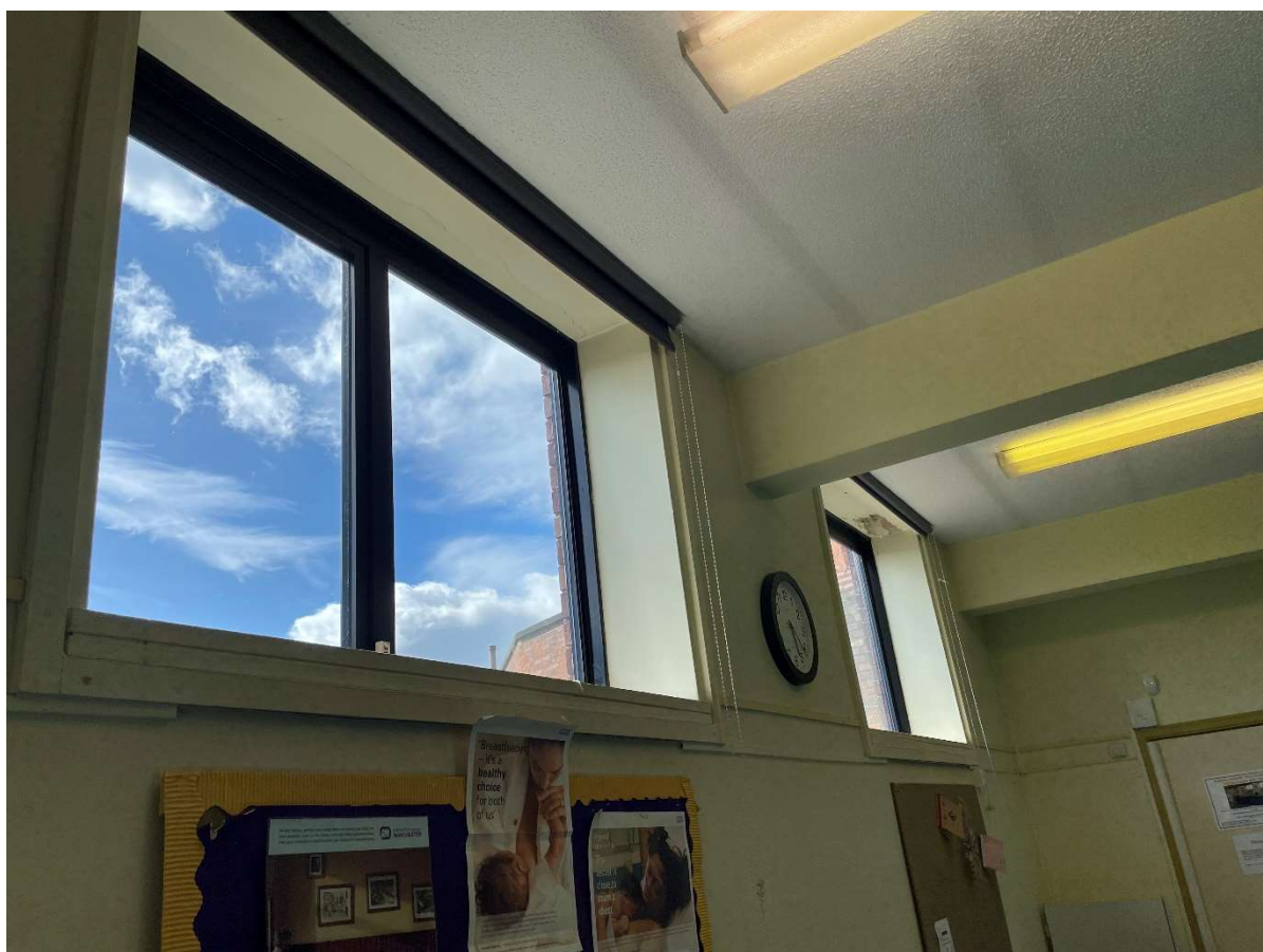
Windows at high level in the west extension wall. Note encased beams and pattern of 'planks' seen on ceiling.
