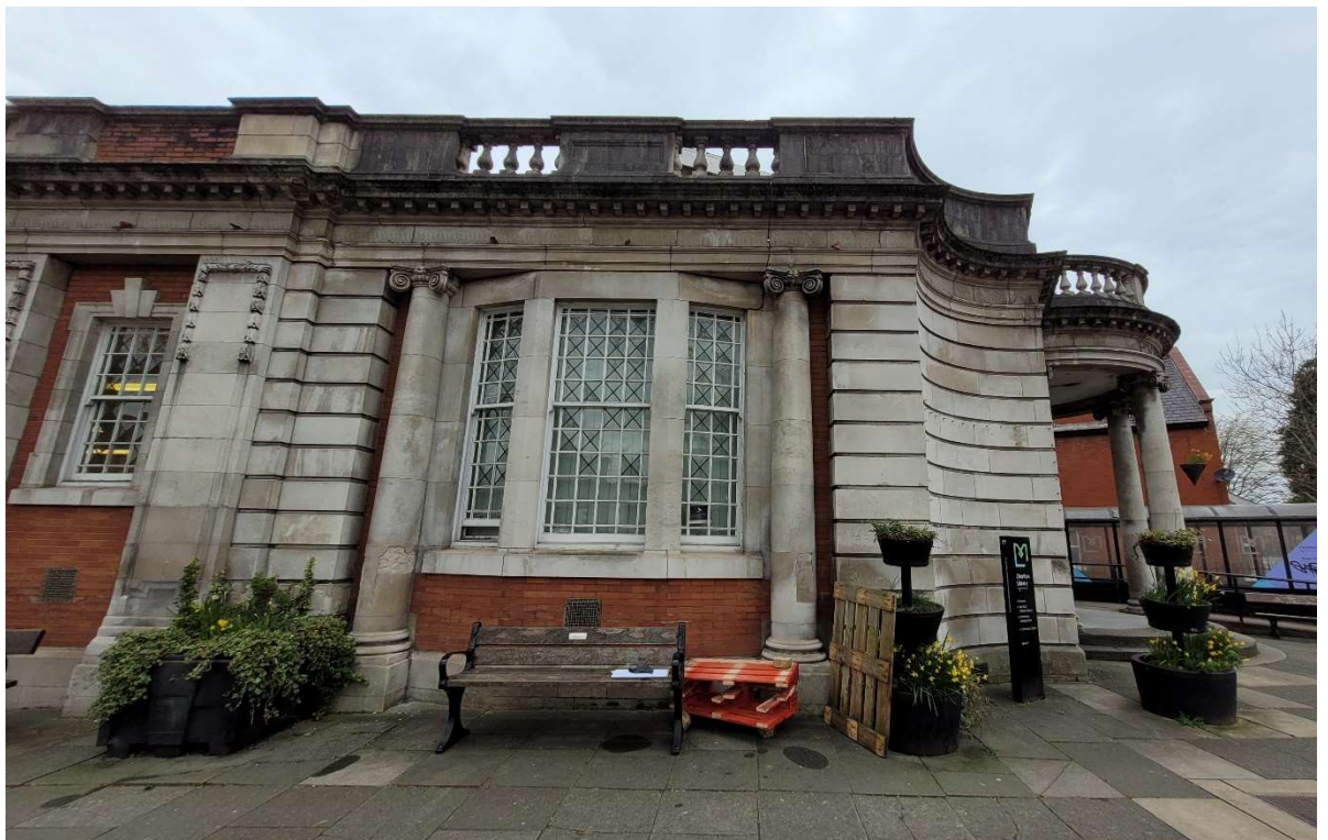
Bay Window to Office, north end of east elevation to Manchester Road
