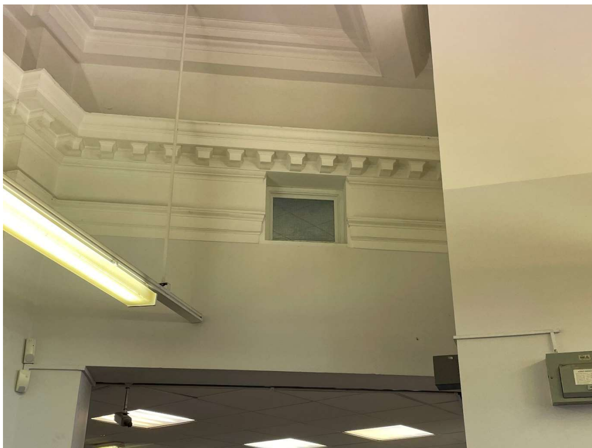
Windows from the gallery into the main volume of the library.
