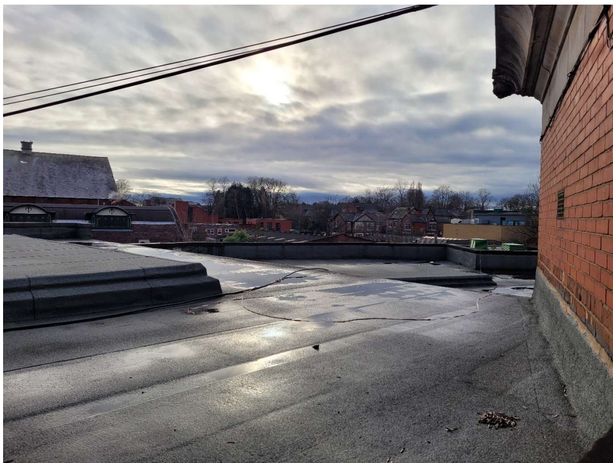
Looking south over the felt roof areas to the rear of the rotunda.
