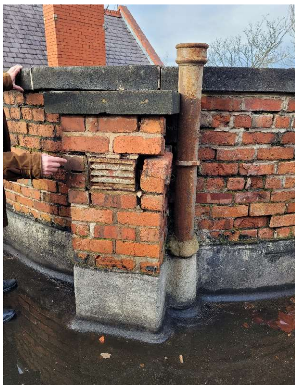
Duct to west of Portico to be rebuilt, and north wall of rotunda from the Portico roof.
