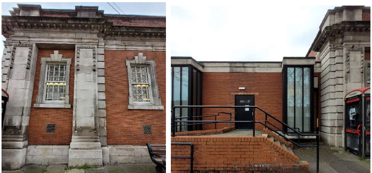
Details at the south end of the Listed Building east wall, and abutment with the unlisted extension.
