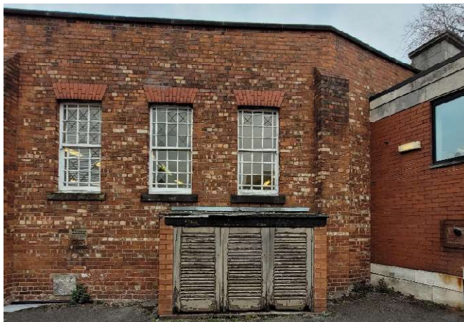
Extension abutment to the south/west walls of the original building. Store doors and roof to be renewed.
