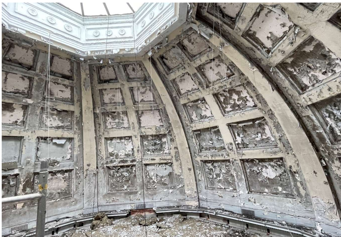
The detail of the Rotunda largely survives above the suspended ceiling in the Staff Room.
