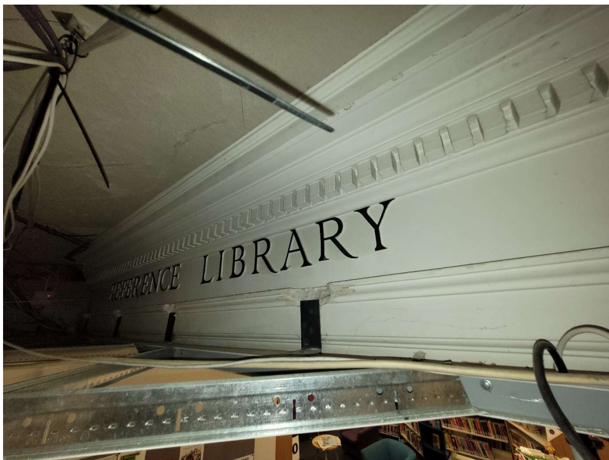
Beneath the original rotunda gallery floor much of the plaster detail remains above the suspended ceiling.
