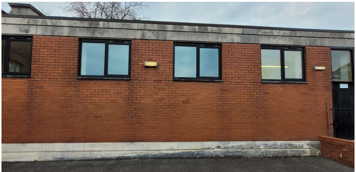
Central section of the extension west wall.
