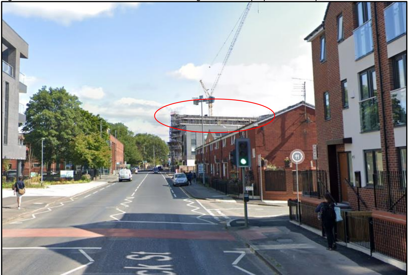
Figure 5.3: Street view from Brunswick Street facing towards the proposed development.
