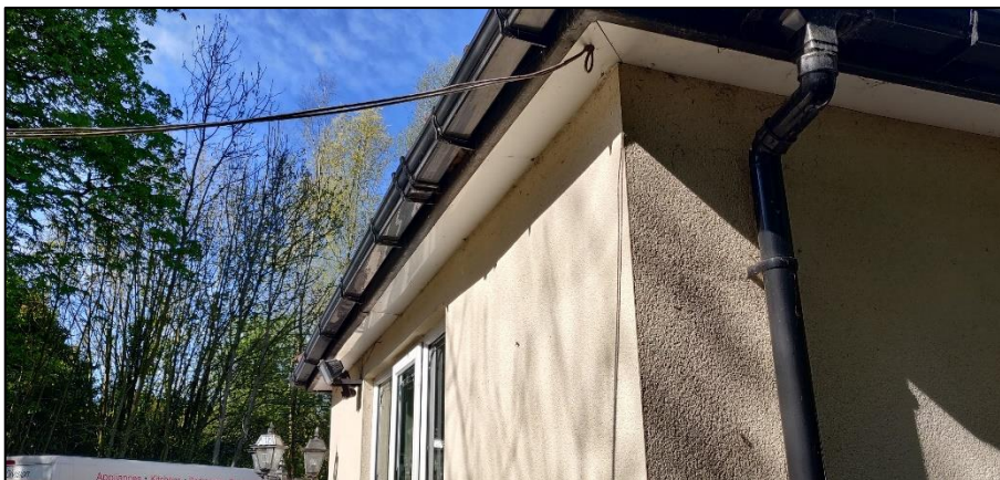
Photograph 2 showing the side elevation of the house
