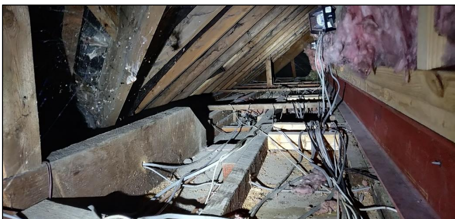
Photograph 5 showing the roof timbers
