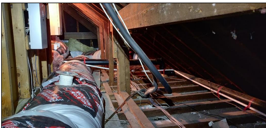
Photograph 6 showing another part of the eaves void
