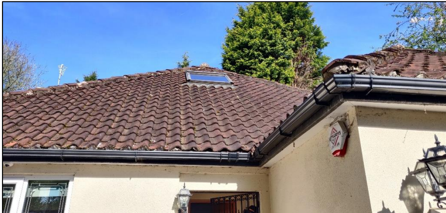
Photograph 3 showing the roof of the property
