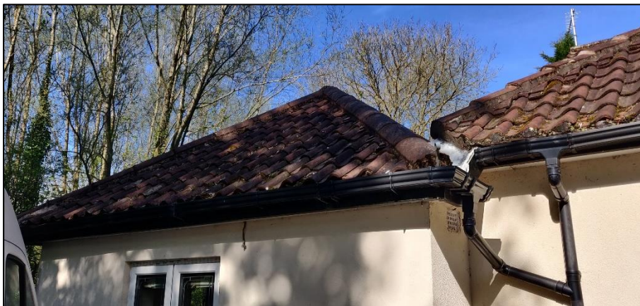
Photograph 4 showing the roof and soffits
